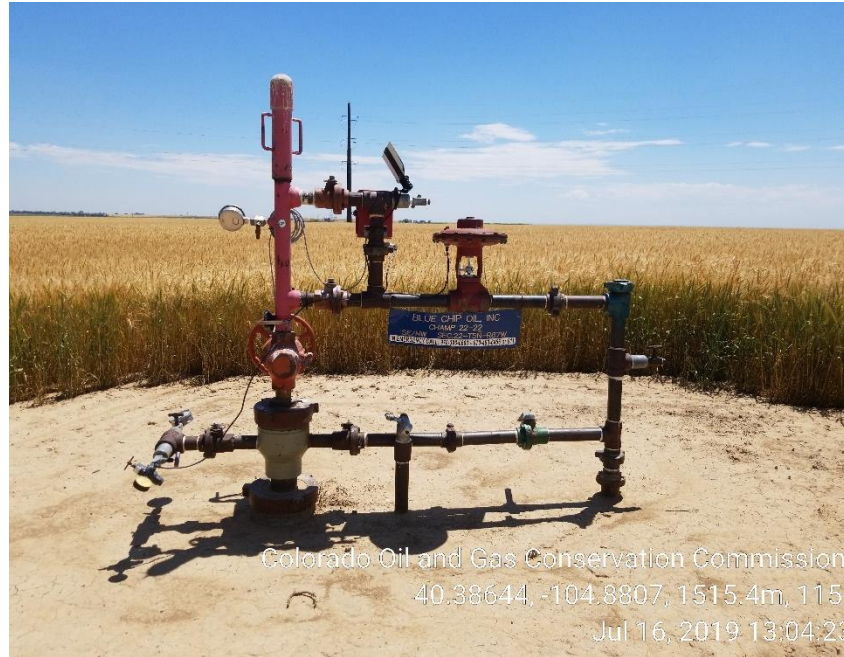
Photo 1: Wellhead; trash removed
