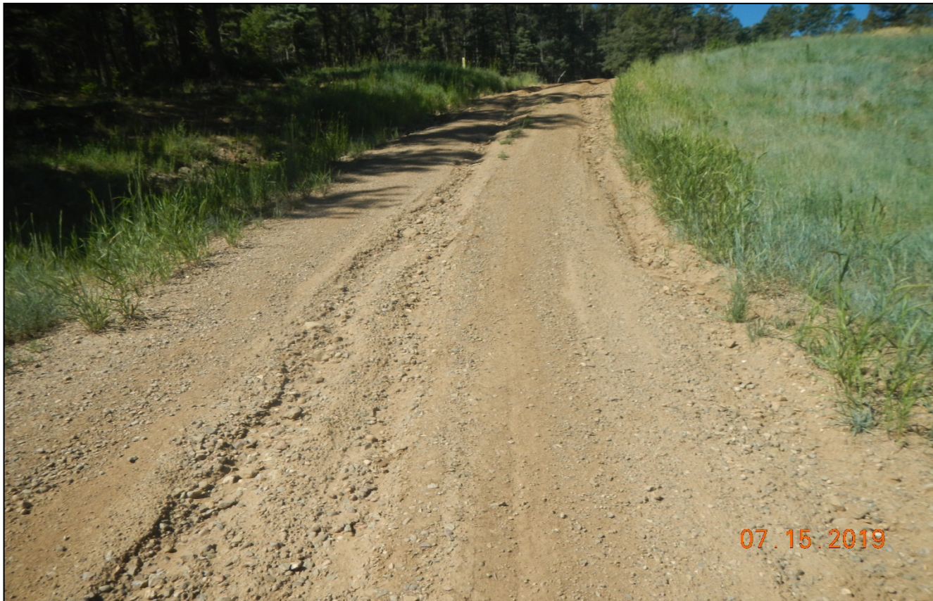
Photo 1. There are vehicle ruts which creates a conveyance for stormwater erosion.
