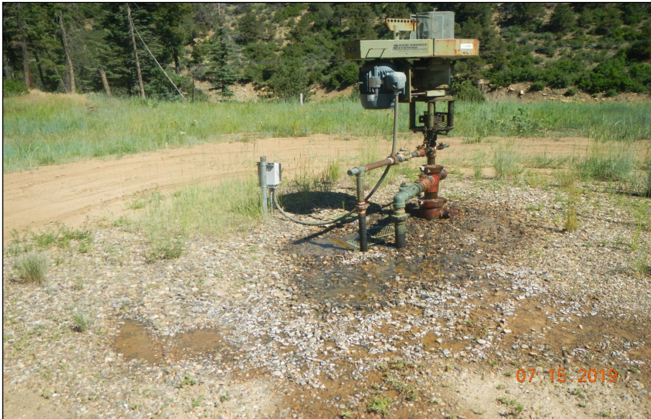
Photo 2. There is a water leak occurring at the wellhead.
