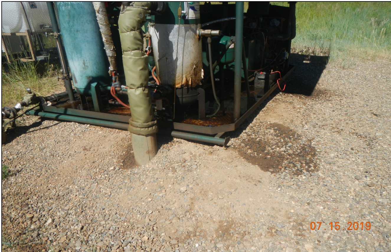
Photo 3. There is oil in the engine skid and staining.
