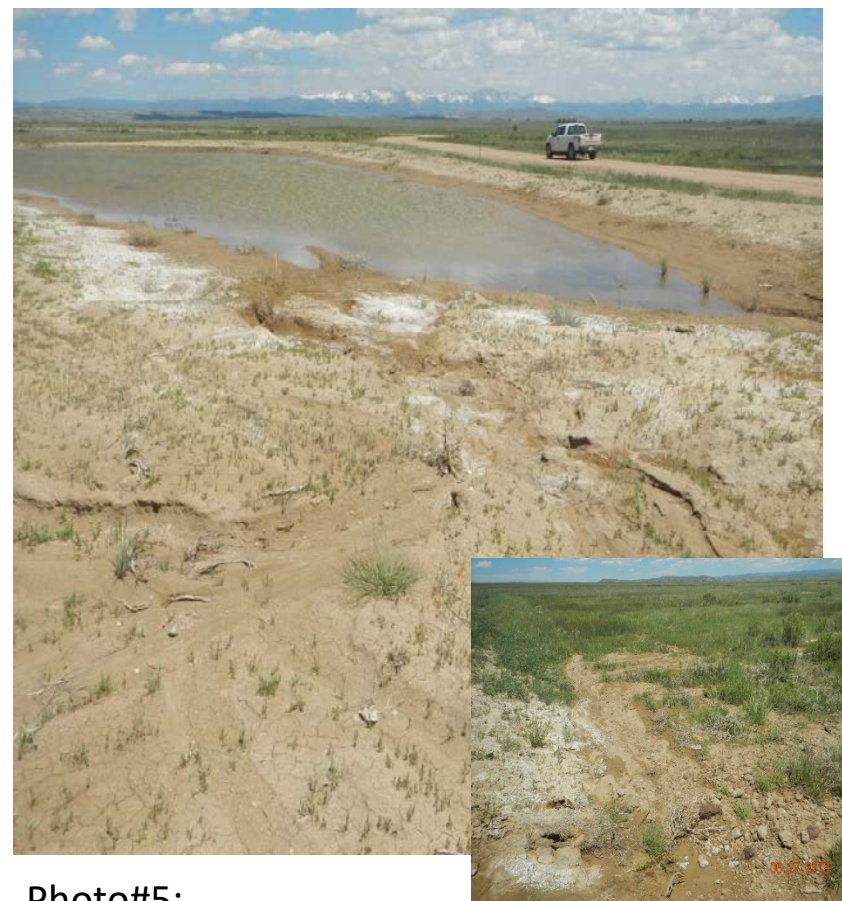
Photo#5: Sediment reservoir & sediment moving off site.
