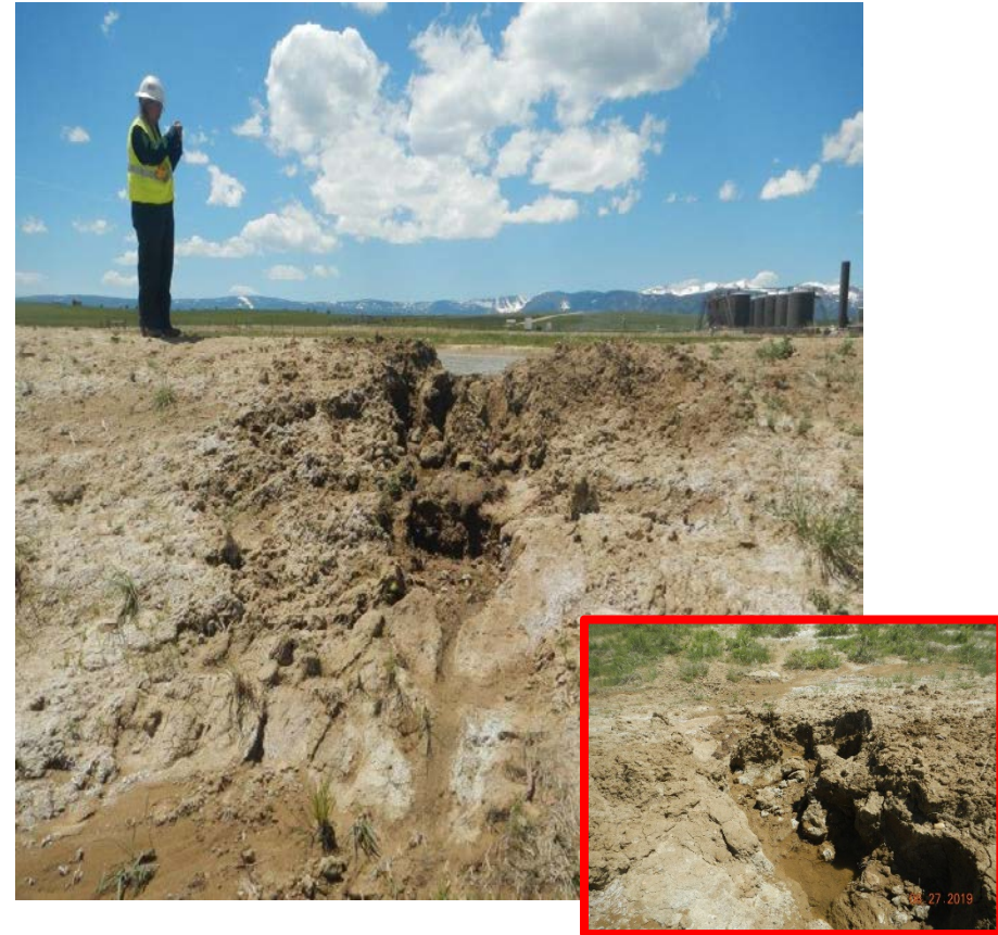
Photo#7: Washout point in reservoir berm
