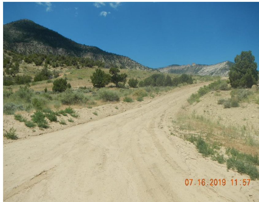
Weeds on access road. Washing and riling of roadway.
