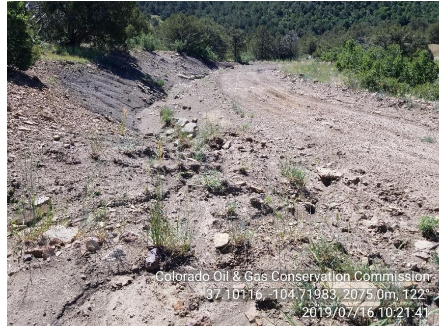
PHOTO 4: ANOTHER IMAGE OF EROSION DOWN GRADE OF BURIED CULVERT
