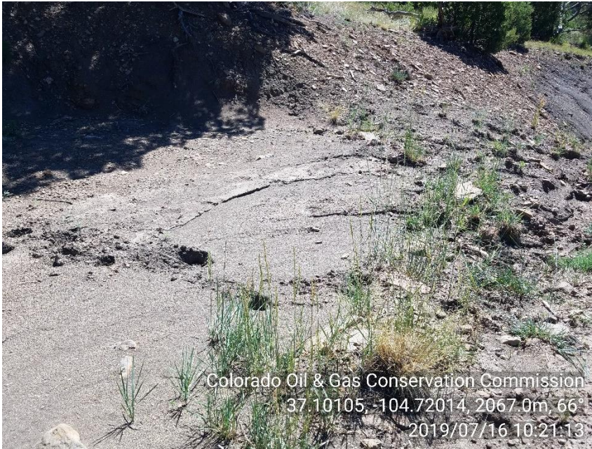
PHOTO 3: CULVERT IS FULL OF SEDIMENT ALLOWING STORMWATER TO ERODE BMP.
