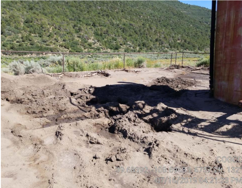
Photo 3. Missing berm.
