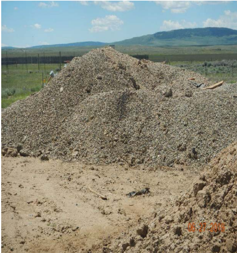
Photo#4: Material piles on site, have trash/debris mixed with material. No BMPs employed on stockpiles.
