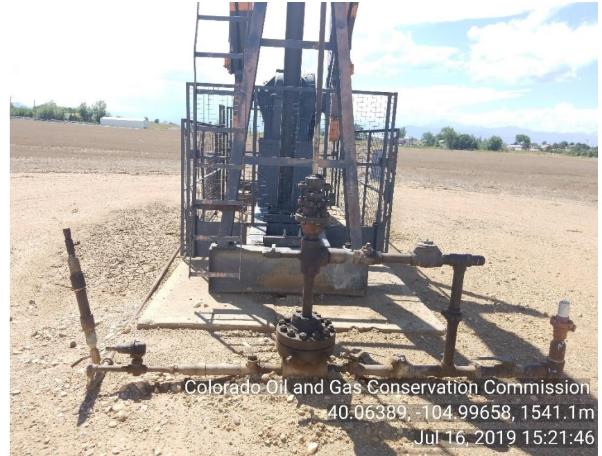
Photo 2 appears all stained soil around PU base and well head has been removed.
