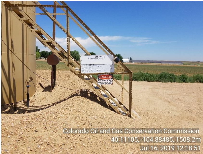
Photo 11 TNK BTRY sign faded not legible.
