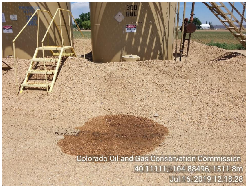
Photo 9 Stained soil from what appears to be from trucks unloading.
