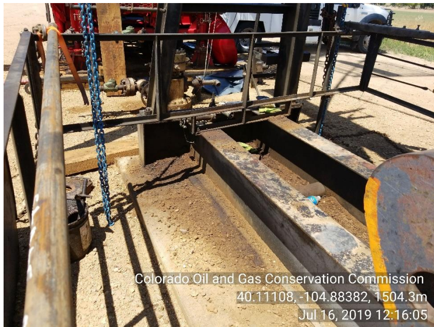
Photo 7 Stained soil in and around PU base
