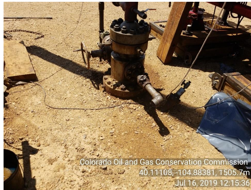
Photo 6 Stained soil around WH
