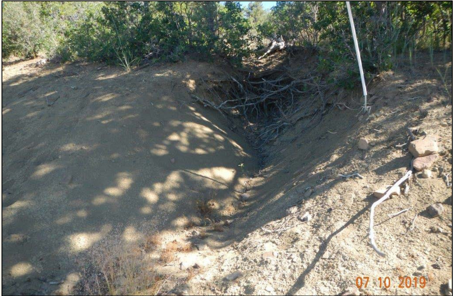
Photo 3. View of erosional channel in northern project area that is eroding the northern cut-slope.
