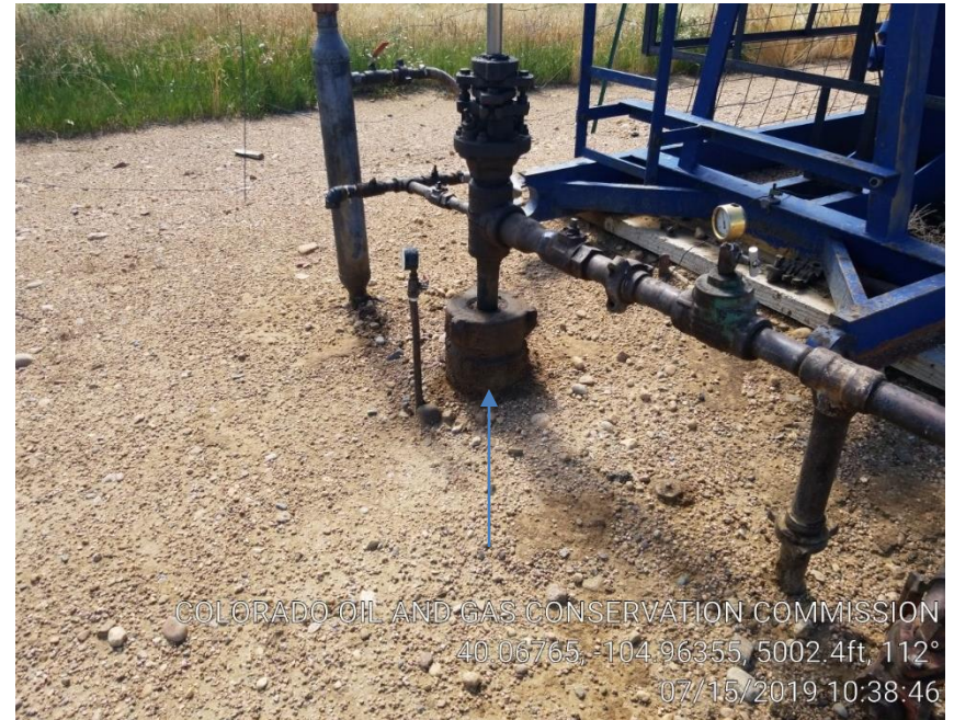
Pic 2 stained soil/possible leak by wellhead
