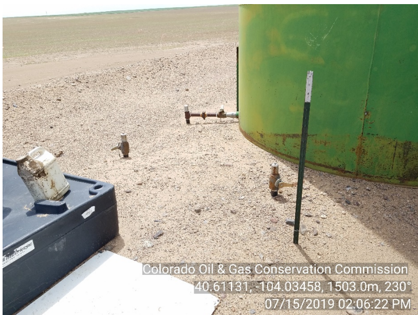
Photo #9 Green 1-1, 1-10 Battery – Crude oil tanks Unused risers SE corner
