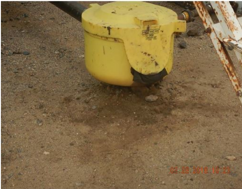
Photo #7 Green 1-1, 1-10 Battery – Crude oil tanks Stained soil at loadout prior insp.
