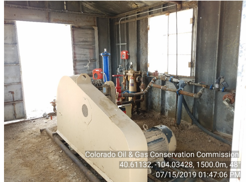
Photo #4 Green 1-1 UIC - Facility Injection Pump
