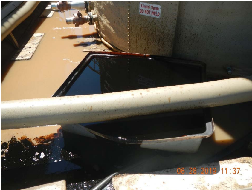
Photo 1. Overflowing stock tank with oily waste inside berm, oily waste in berm.
