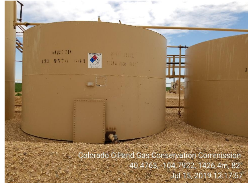
Photo 4: Labeling faded on crude oil tank.
