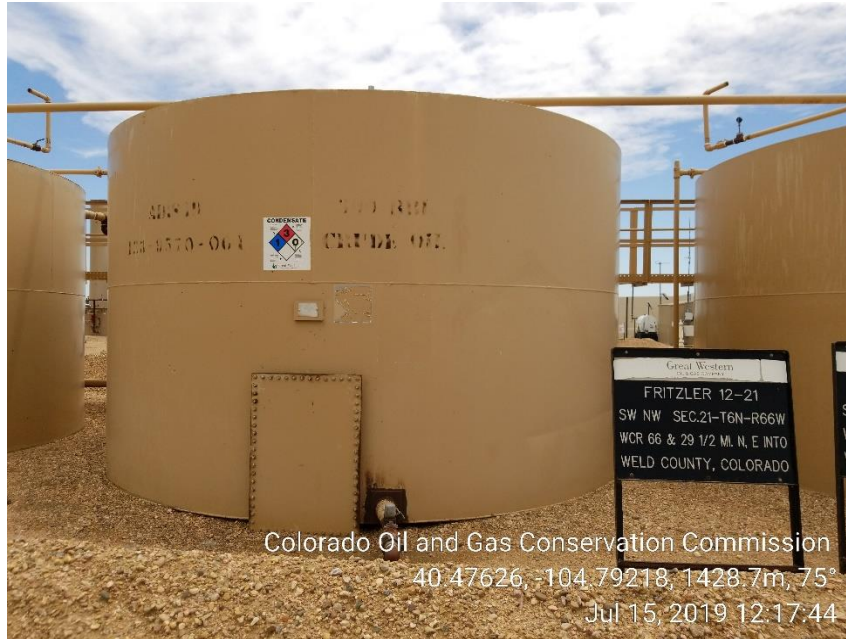
Photo 3: Labeling Faded on crude oil tank.
