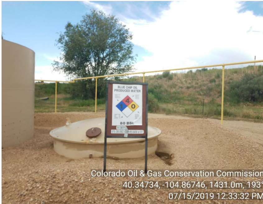
Produced water vault placarding at tank battery
