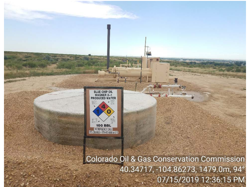
Produced water vault placarding at separator
