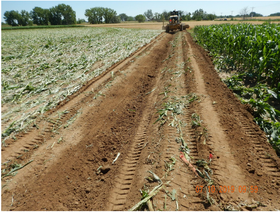
Photo 1. Photo taken from the southern Location, facing East. Photo illustrates Operator was in-process of installing the perimeter BMP (ditch and berm) at the time of my inspection.
