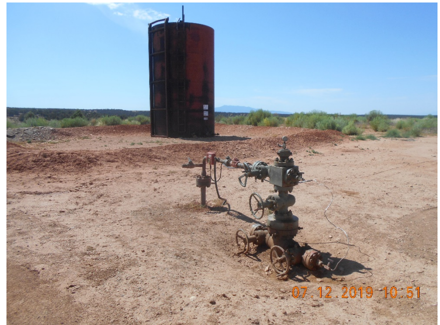
Injection wellhead. Tank Battery.
