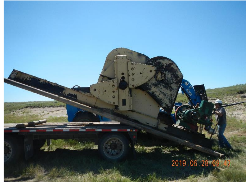
Photo 6: Loading the pumping unit base onto the trailer.
