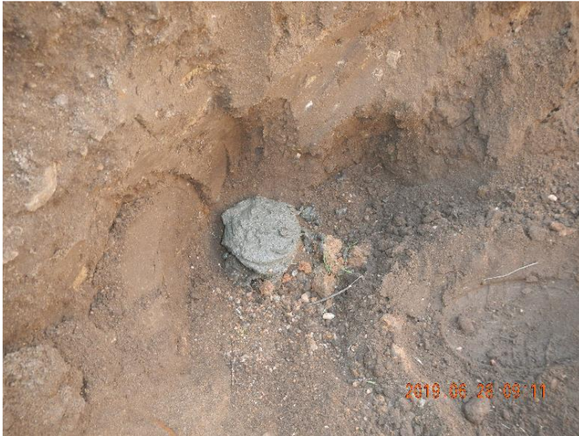
Photo 5: Cement plugged and abandoned wellhead flow line.
