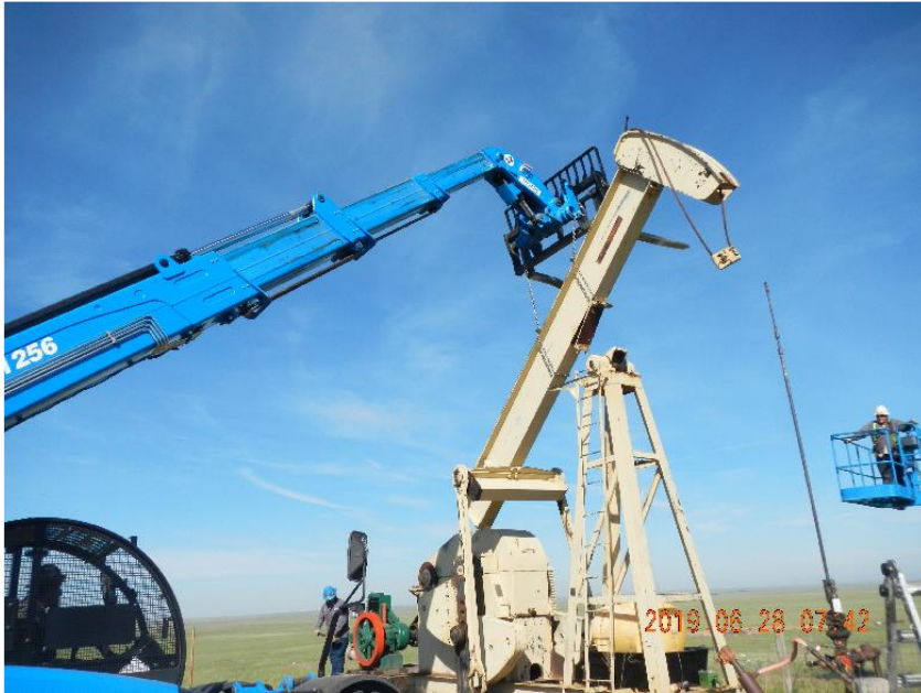
Photo 3: Removing the horsehead, walking beam and pitman arms from pumping unit.
