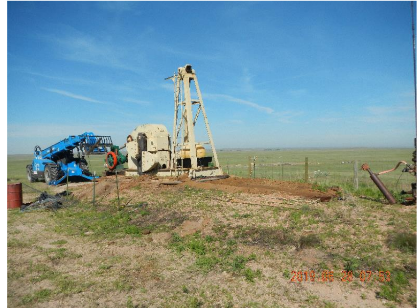
Photo 4: Sliding pumping unit base from wellhead.
