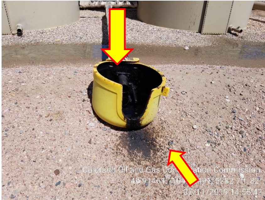
Photo 5 – Loadline Bucket, stained soil.
