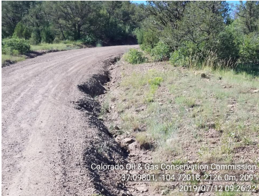
PHOTO 3: AREA OF EROSION ON WEST SIDE OF ROW NORTH OF LOCATION TOWARD THE BOTTOM OF THE HILL. REPAIR EROSION AND REPAIR OR INSTALL BMP'S TO PREVENT EROSION AND COMPLY WITH RULE 1002.f. CA DATE 8/12/19
