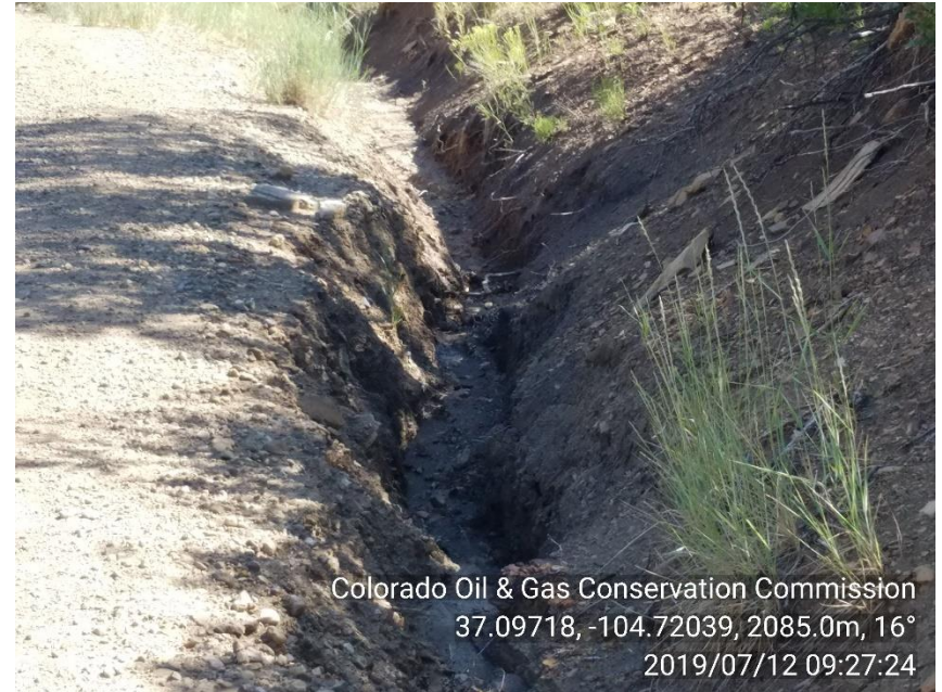
PHOTO 4: AREA OF EROSION ON EAST SIDE OF ROW NORTH OF LOCATION TOWARD THE BOTTOM OF THE HILL. REPAIR EROSION AND REPAIR OR INSTALL BMP'S TO PREVENT EROSION AND COMPLY WITH RULE 1002.f. CA DATE 8/12/19
