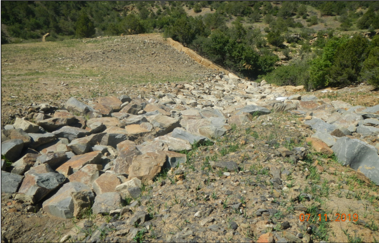
Photo 5. Rock rip/rap is installed at the lower part of the location for outlet protection.
