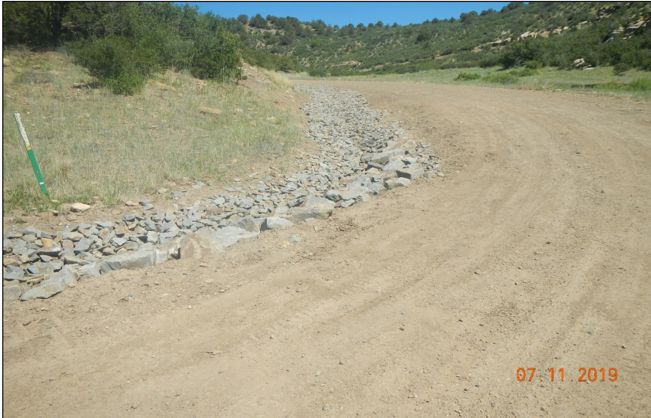
Photo 4. Rip/rap has been installed along the side of the road where erosion was occurring.
