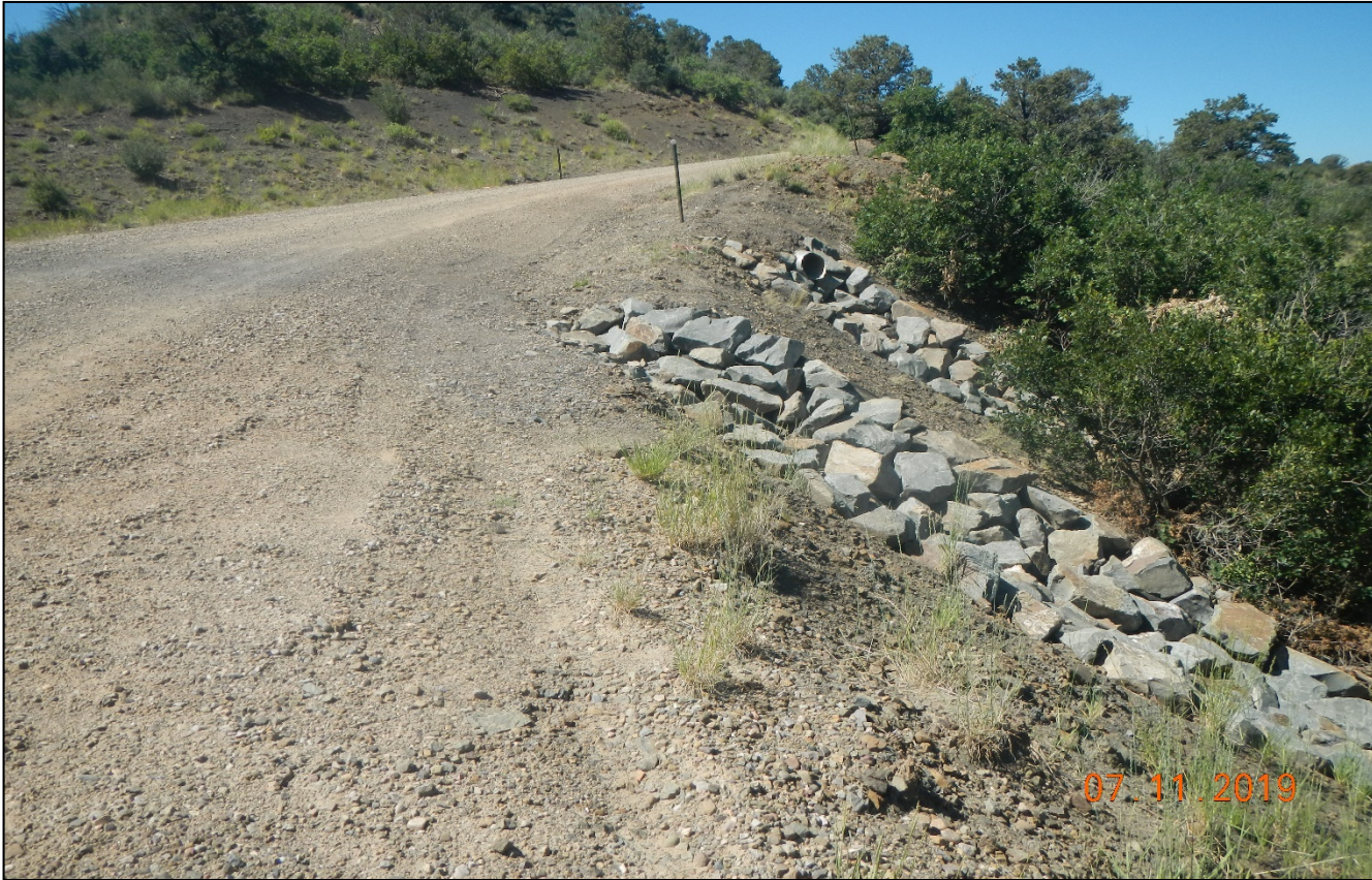
Photo 2. Facing along the main road. Rock rip/rap has been installed as outlet protection at numerous culvert outlets.
