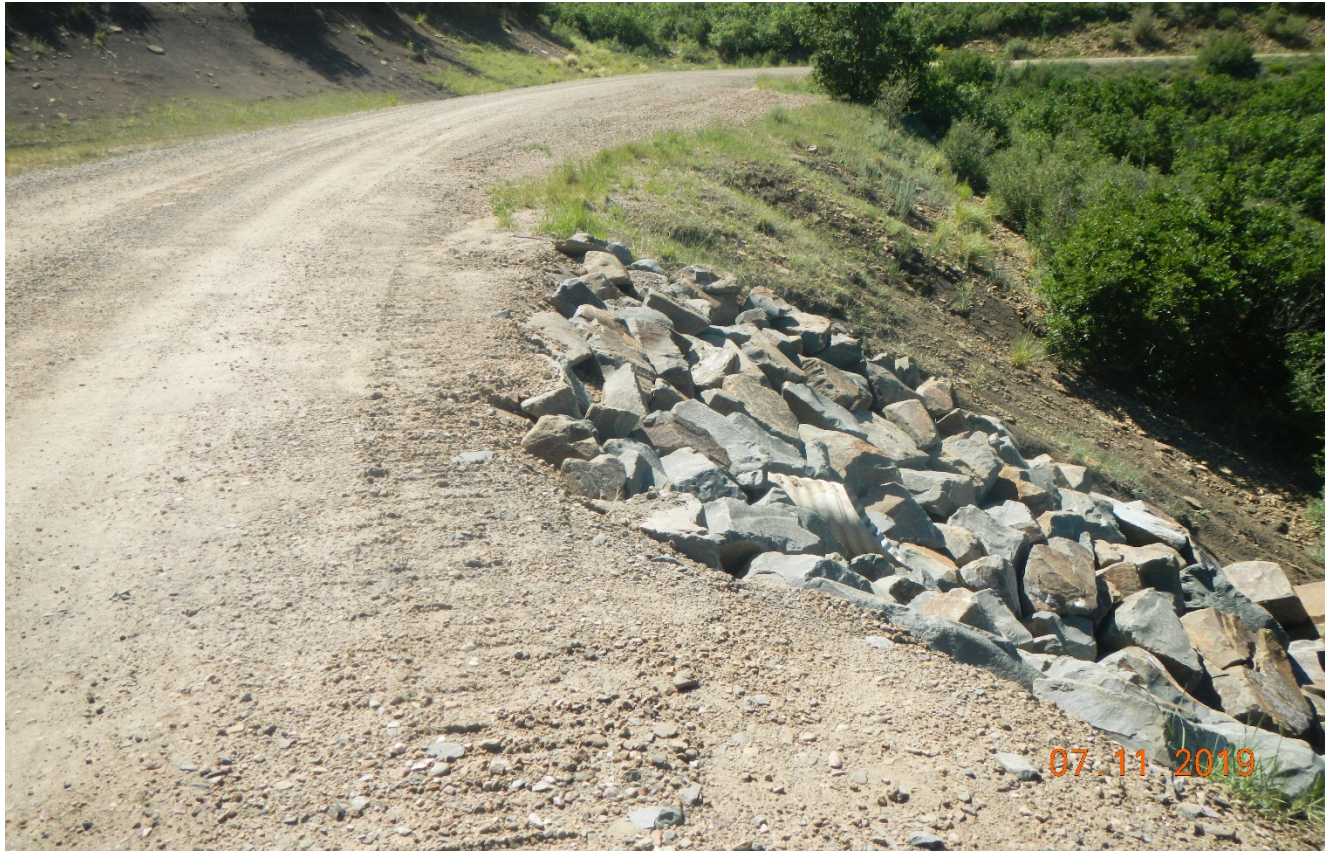
Photo 1. Facing along the main road. Rock rip/rap has been installed as outlet protection at numerous culvert outlets.
