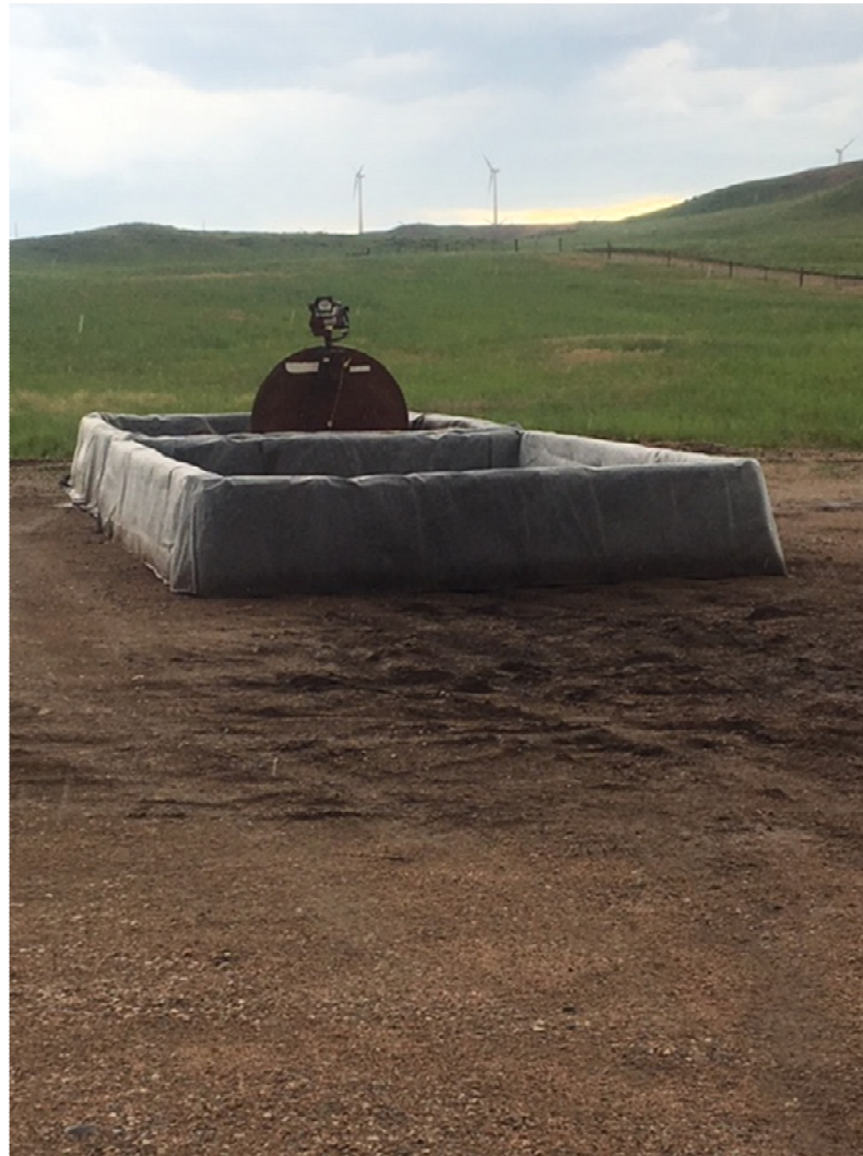
Photo 1 – Diesel Fuel Containment
