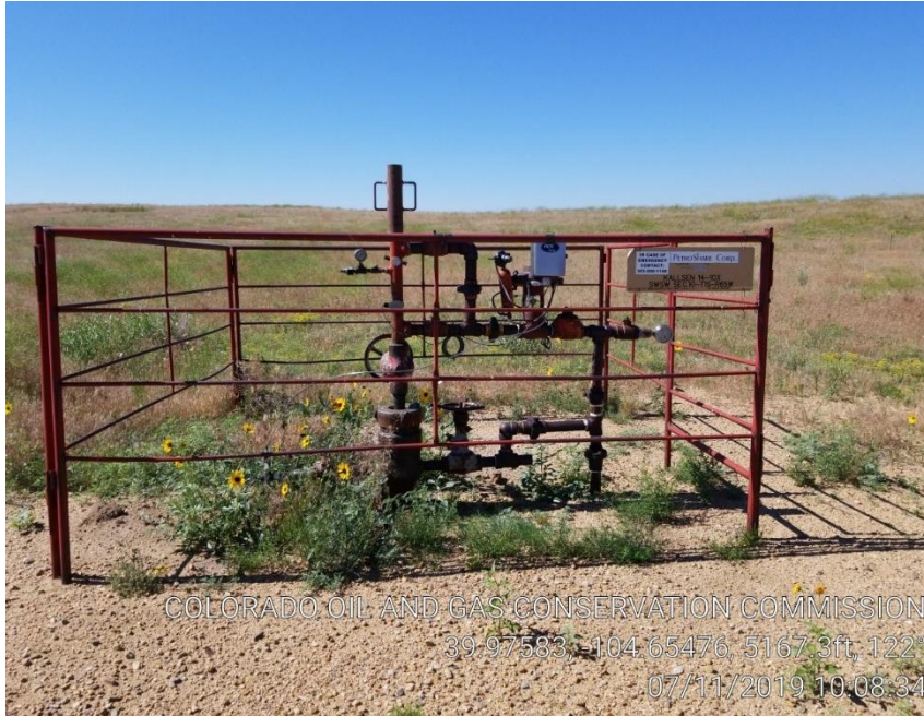
Pic 1 wrong operator name on sign
