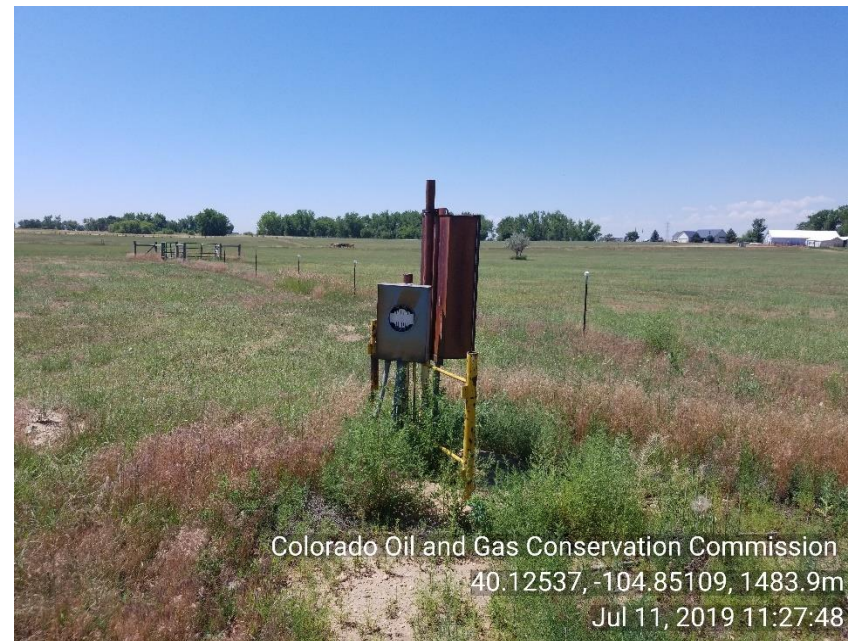
Photo 4 Unused equipment: Electric panel and breaker box, meter has been removed.
