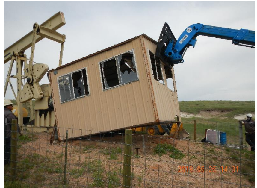
Photo 2: Removing the prime mover shed.
