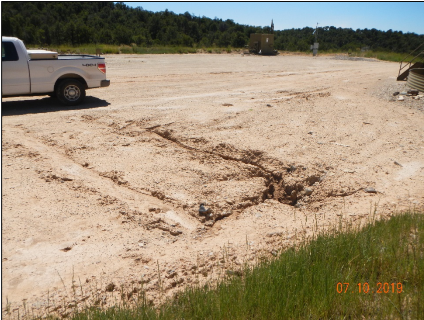
Photo #9 Erosion leading to a hole on location
