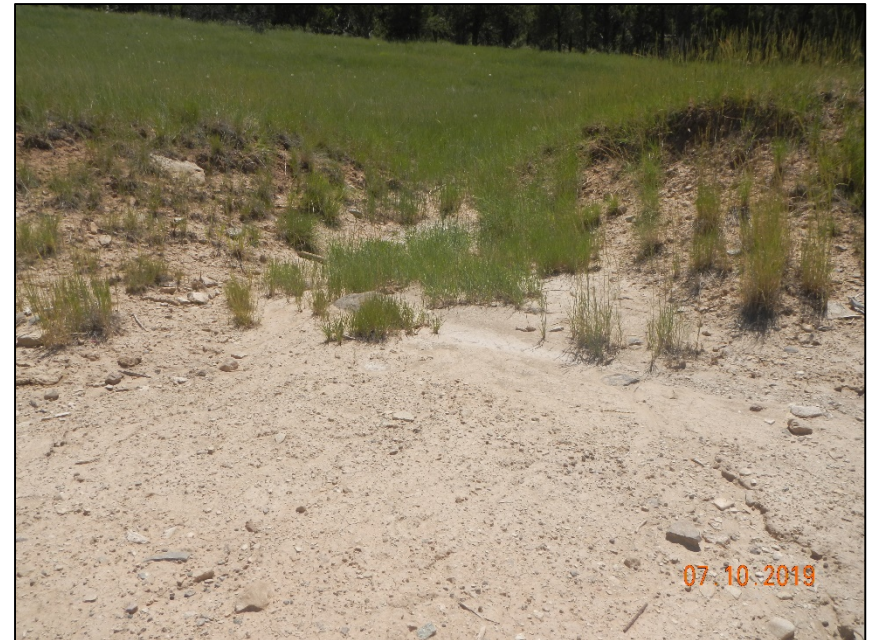
Photo #10 Storm water BMP need maintenance. Drain is full of sediment.
