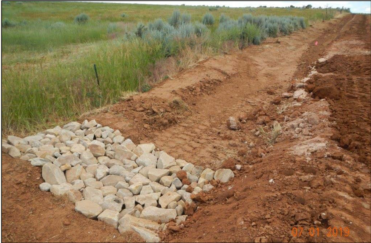
Photo 4. View of rock check along access road and compacted berm in place.
