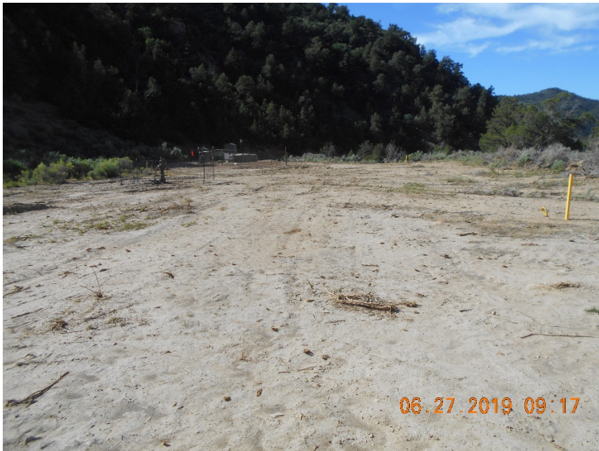
Location overview looking S.
