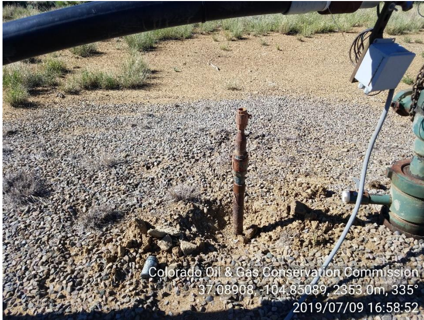
PHOTO 5: UNUSED EQUIPMENT (2" RISER NEAR WELLHEAD). REMOVE UNUSED RISER IN ACCORDANCE WITH NTO AND WITH RULE 603.f. CA DATE 10/9/19
