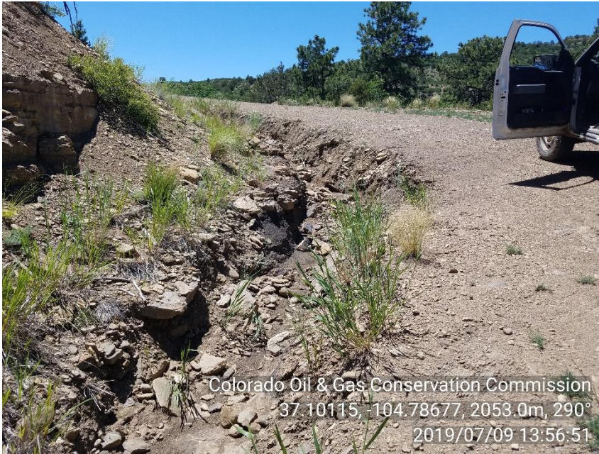
PHOTO 3: EROSION IN DITCH ALONG ACCESS ROAD NORTH OF LOCATION. REPAIR EROSION, INSTALL BMP'S AND MAINTAIN IN ACCORDANCE WITH 1002.f. CA DATE 8/9/19.
