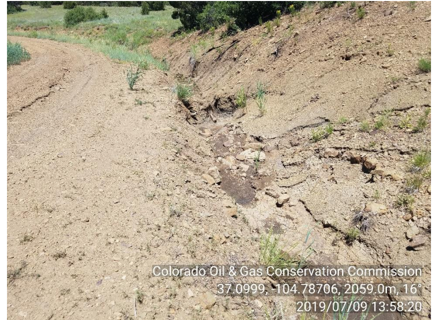
PHOTO 4: EROSION IN DITCH ALONG ACCESS ROAD NORTH OF LOCATION. REPAIR EROSION, INSTALL BMP'S AND MAINTAIN IN ACCORDANCE WITH 1002.f. CA DATE 8/9/19.
