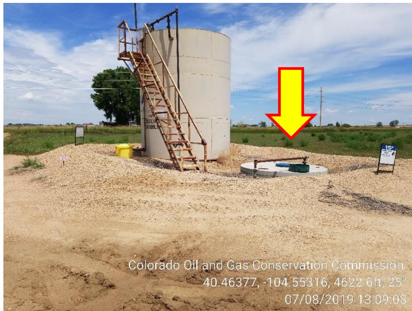
Photo 1 – Tank Battery, inadequate berm height
