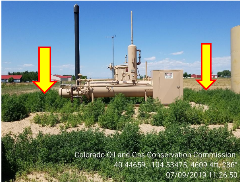
Photo 1 – Separator, overgrown weeds on the entire location
