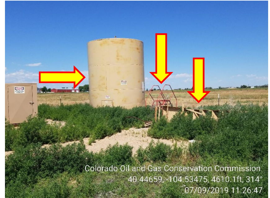
Photo 2 – Tank Battery , overgrown weeds on the entire location. Unused Tank, stairs, and walk over stairs
