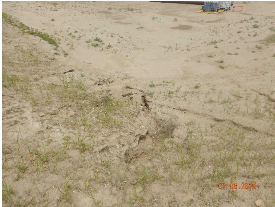
Photo 4: Photo taken from the southeast corner of the location, facing northwest. Photo shows erosion degradation on slopes and sediment deposition has filled in the stormwater ditch.
