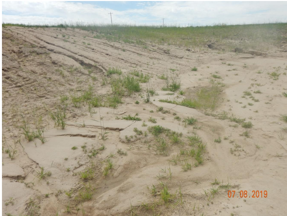
Photo 2: Continued from photo 1. Photo shows erosion degradation on slopes and sediment deposition has filled in the stormwater ditch.
