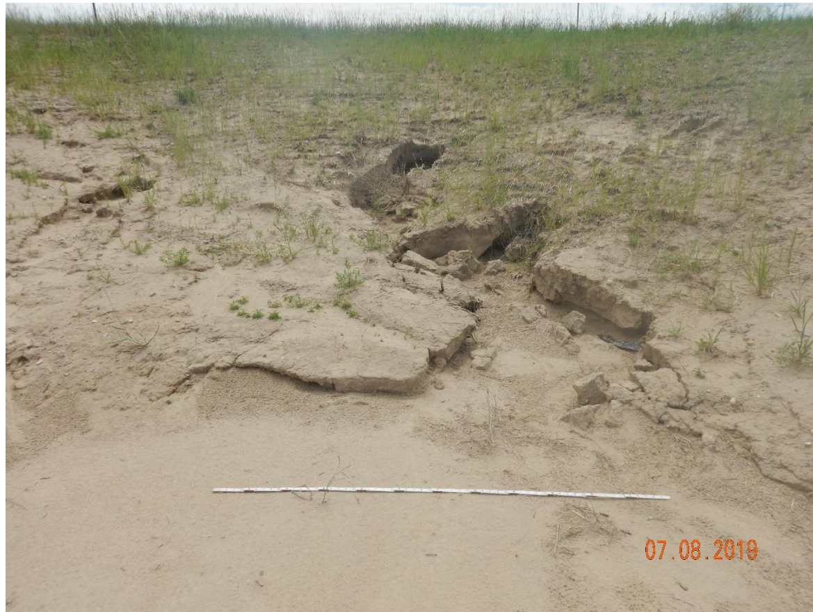
Photo 3: Continued from photo 1. Photo shows erosion degradation on slopes and sediment deposition has filled in the stormwater ditch. 6 foot measuring stick for reference.
