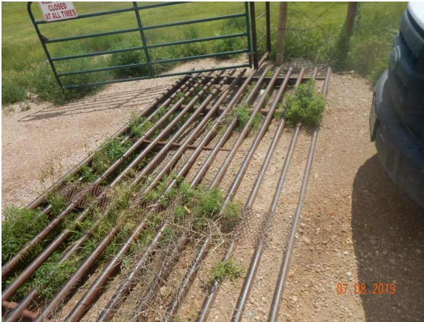
Photo 1: Photo taken from the access road. Photos 1-3 show cattle guards BMPs are filling with sediment. Advise maintenance.
