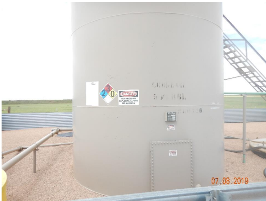
Photo 13: Photo shows labelling on tanks beginning to fade.
