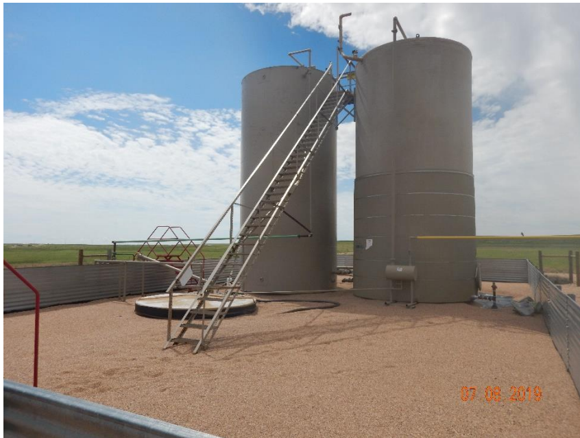
Photo 11: Photo of tank. Two 500 bbl AST, 1 crude, 1 PR water
