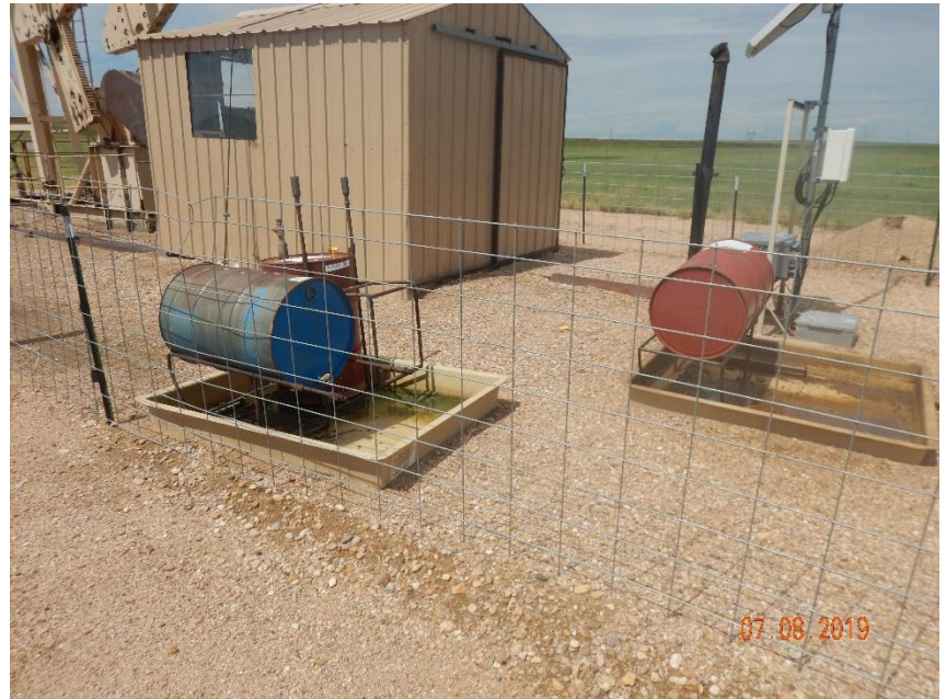
Photo 8: Photo shows barrels within secondary containment.
