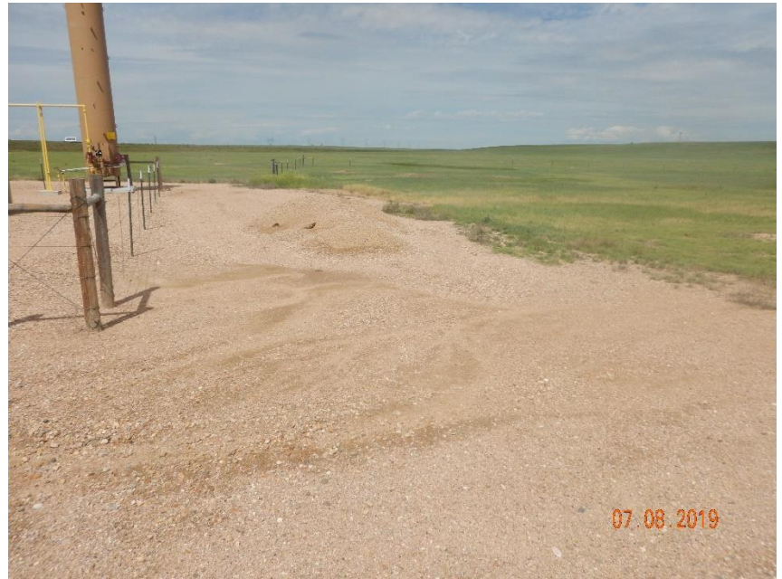
Photo 4: Photo taken from the east end of the battery. Photo shows stormwater erosion degradation.
