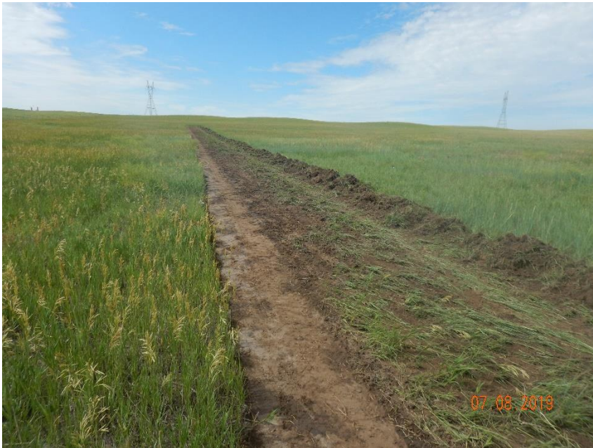
Photo 1: Photo taken from the east end of the location, facing south. Photos 1-4 provide an overview of the location from south, southwest, northwest to north. Photos show operator has delineated the perimeter of the location in preparation for surface roughening and a perimeter ditch.
