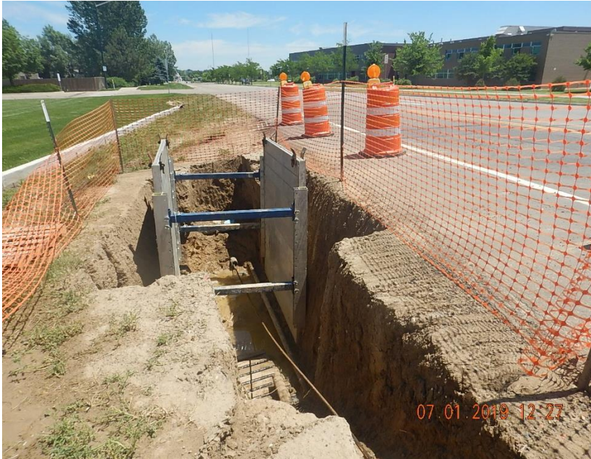
View of second excavation approximately 1250' west of spill ID #463820. An attempt to install a 2" HDPE pipe via slip line was unsuccessful. View east/ photo date 7/1/19
