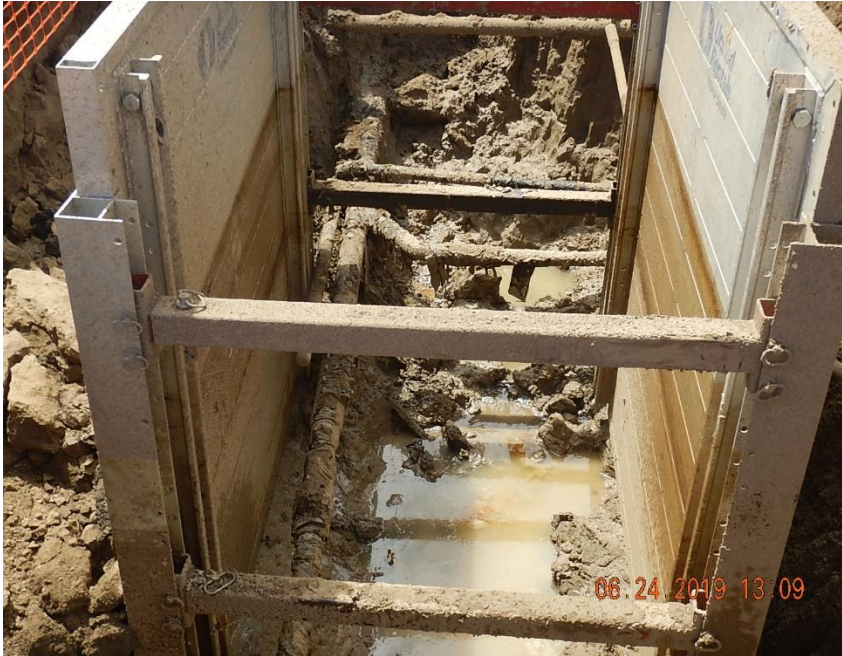
View of flowlines exposed in excavation; bolted clamp can be seen on 3" consolidation flowline. Photo date 6/24/19.
