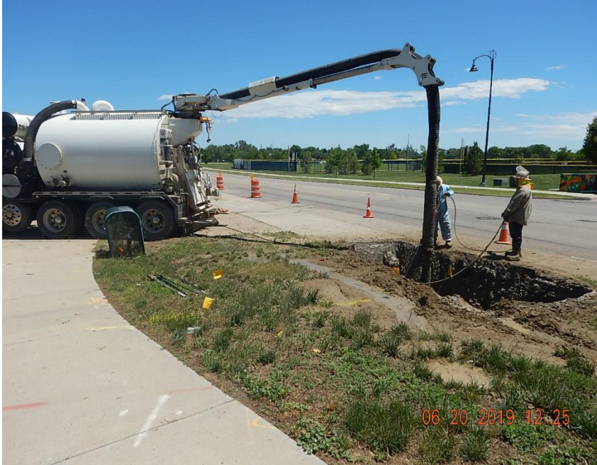
Hydro-excavation work being completed by KPK contractors on 6/20/2019. View looking east on Tipple Parkway.
