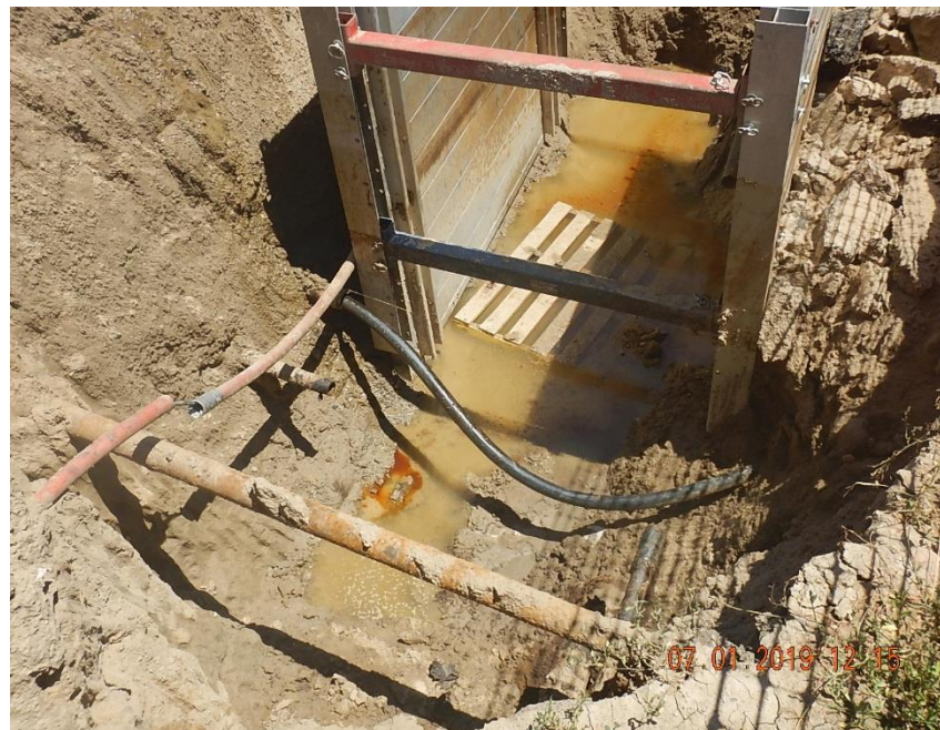
View of excavation and flowline repair/ replacement work in progress. Note: free product (crude oil) is present at trench bottom (on water). Photo taken 7/1/2019
