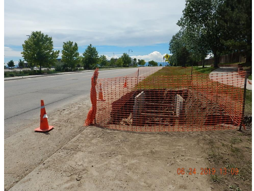
Excavation (fenced) with trench box installed on 6/24/2019. View looking west on Tipple Pkwy.
