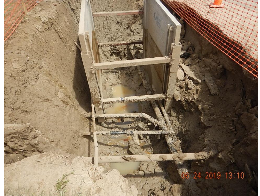
View of flowlines exposed (at spill Id #463820) in excavation. Flowlines tie in to crude oil and gas consolidation lines. Note: Marked utilities (non KPK/ via 811 call) are also present in the excavation.
