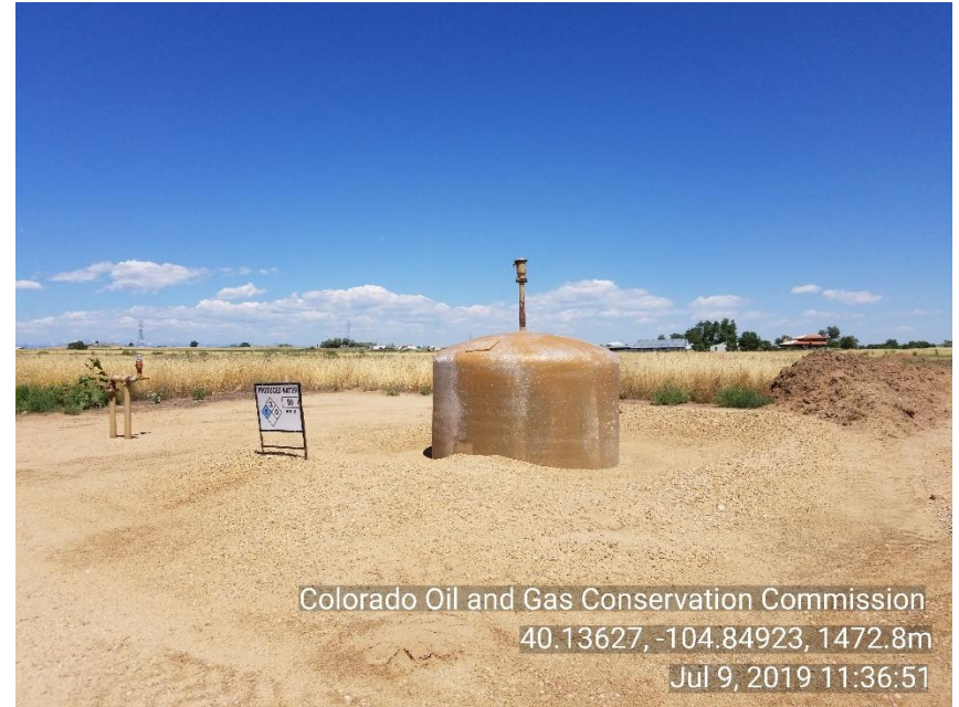
Photo 4 50BBL produced water tank.
