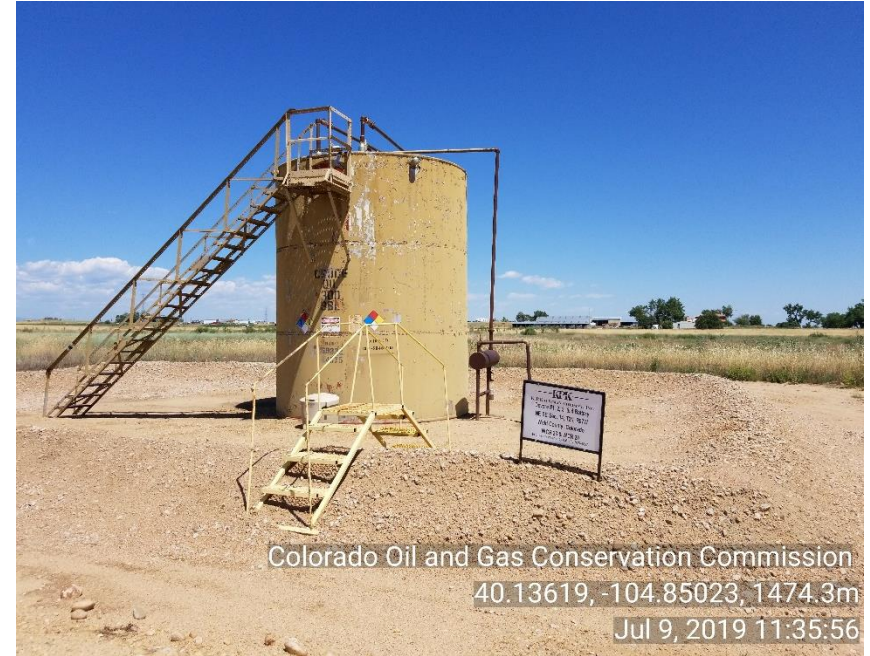
Photo 2 Crude oil tank.
