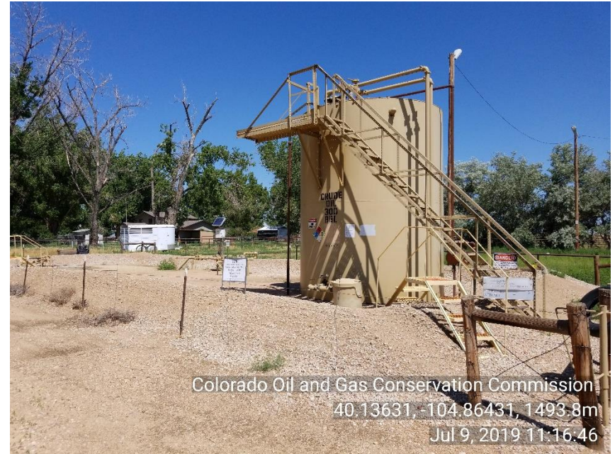
Photo 4 TNK BTRY. I appears berm has been repaired.
