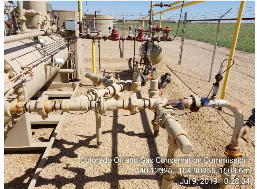
Photo 4 inlet flow lines to separator locked closed.
