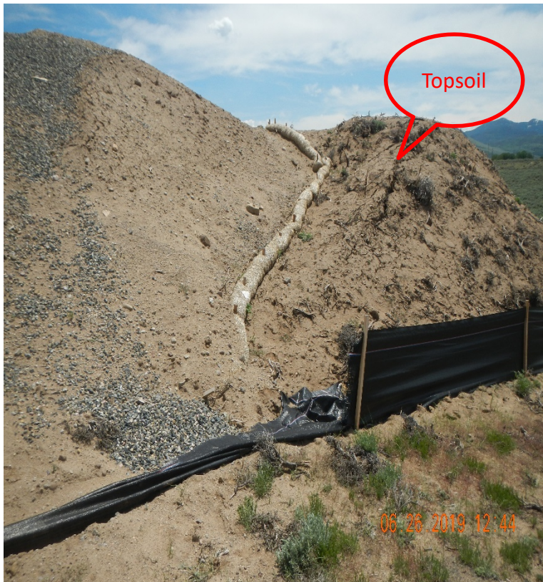
Photo#6: Slopes/ topsoil stockpile are not stabilized, resulting in erosion, sediment migration and degradation.
