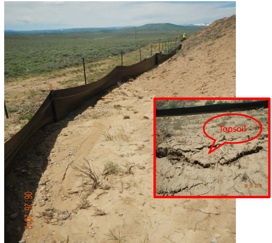
Photo#7: Slopes/topsoil stockpile are not stabilized, resulting in erosion, sediment migration and degradation.
