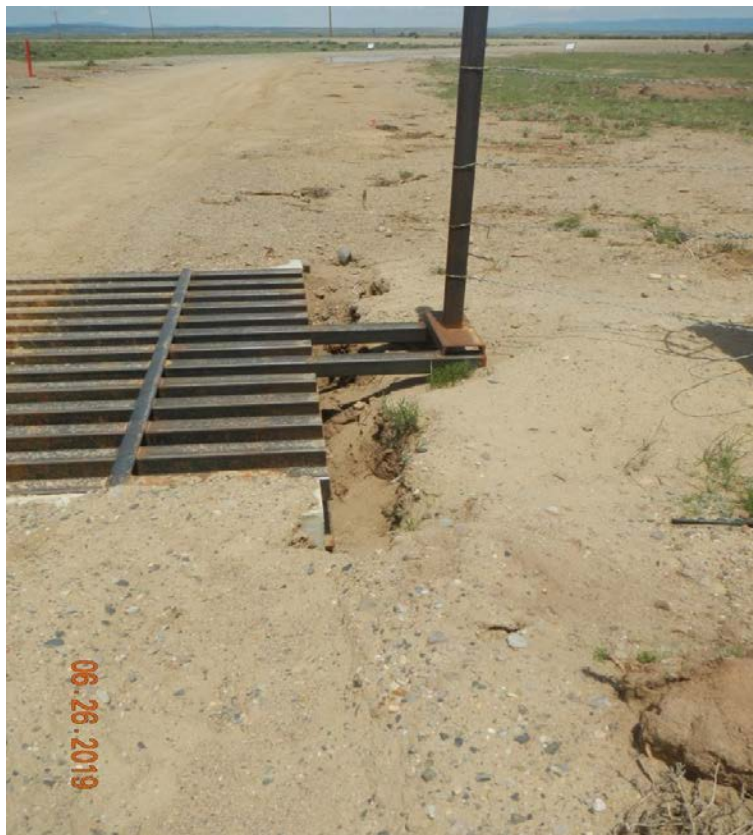
Photo#10: Absence of BMPs at entries and along access road.
