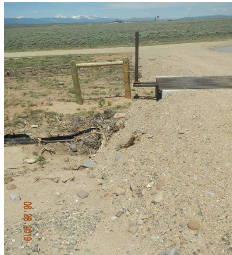
Photo#11: Absence of BMPs at entries and along access road.
