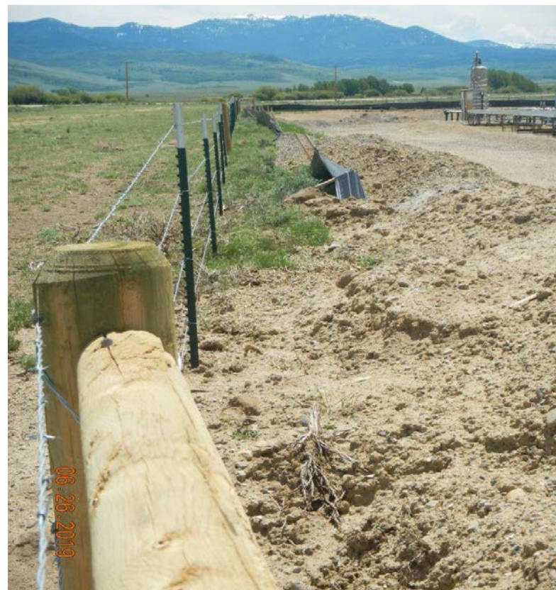
Photo#3: Silt fence buried.
