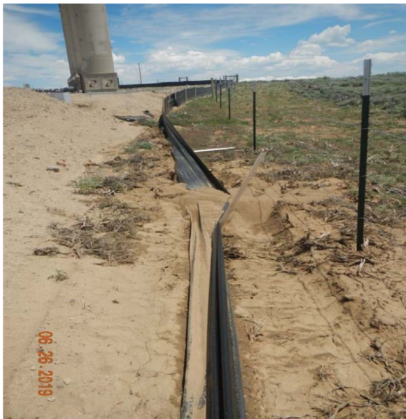
Photo#2: Silt fence overwhelmed.
