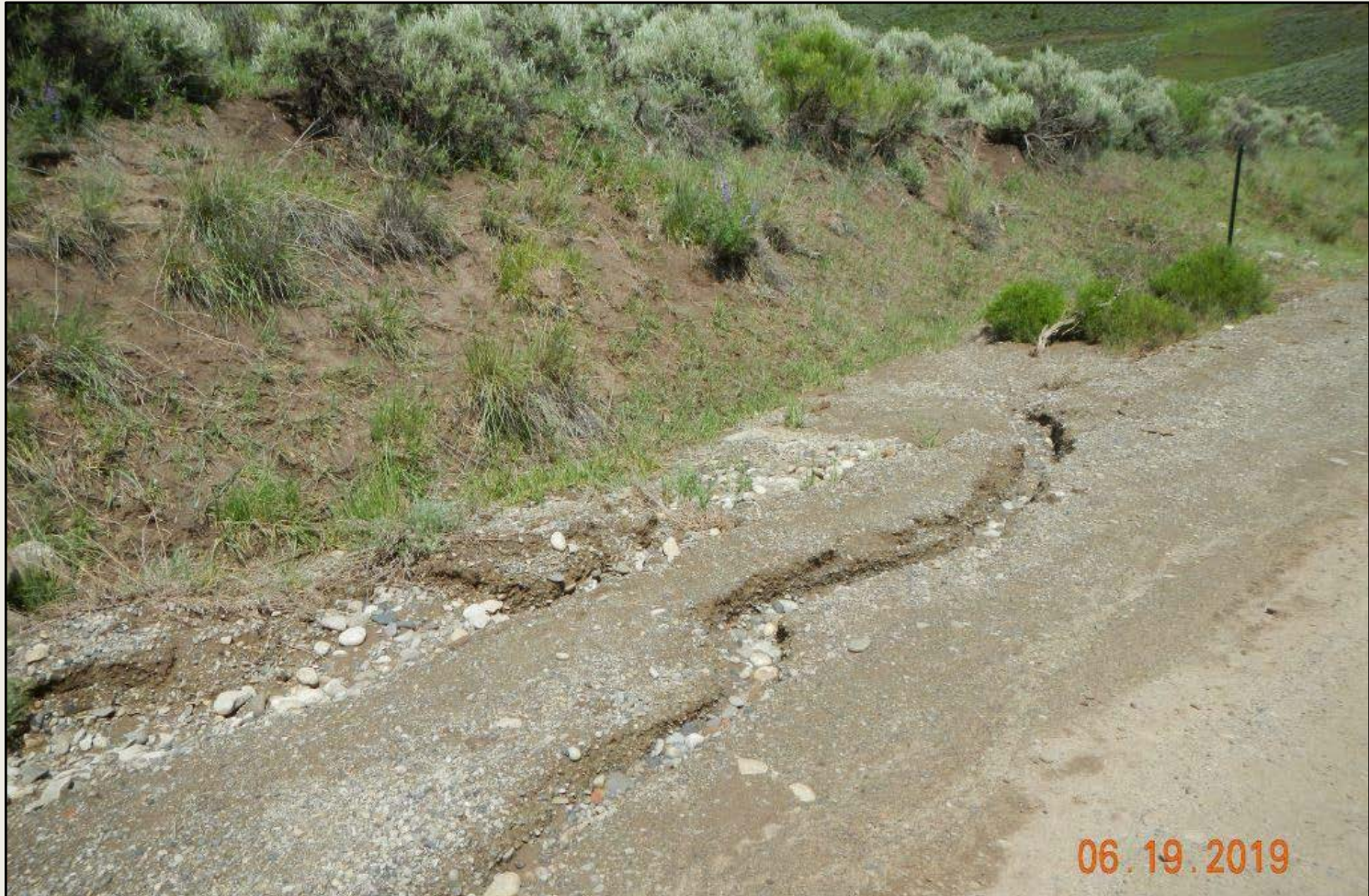
Photo 2. View of erosional channeling and down-cutting along the access road.
