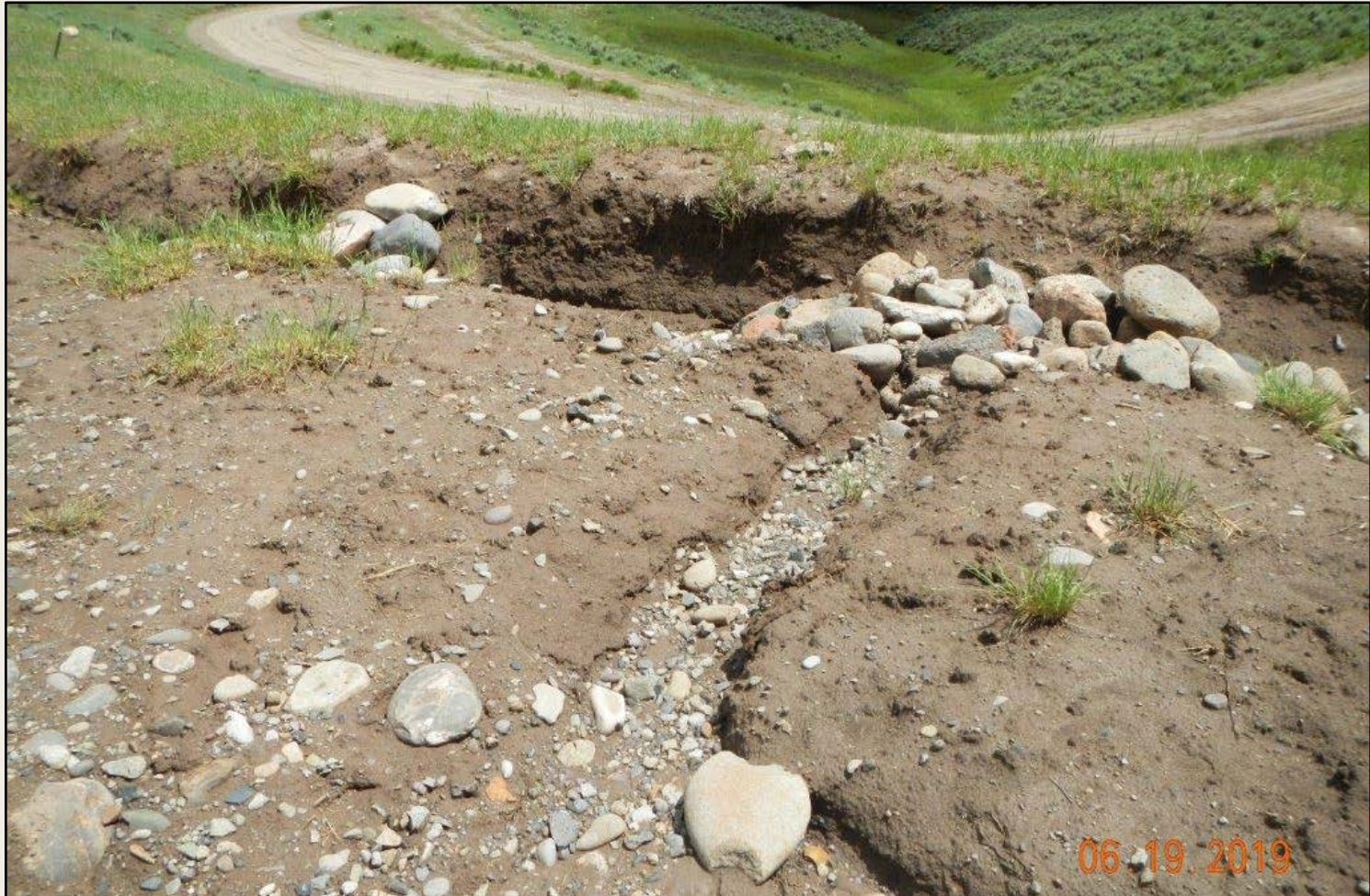
Photo 2. View of erosional channeling and downcutting along the southern edge of the project area. Rock checks do not appear to be functioning.
