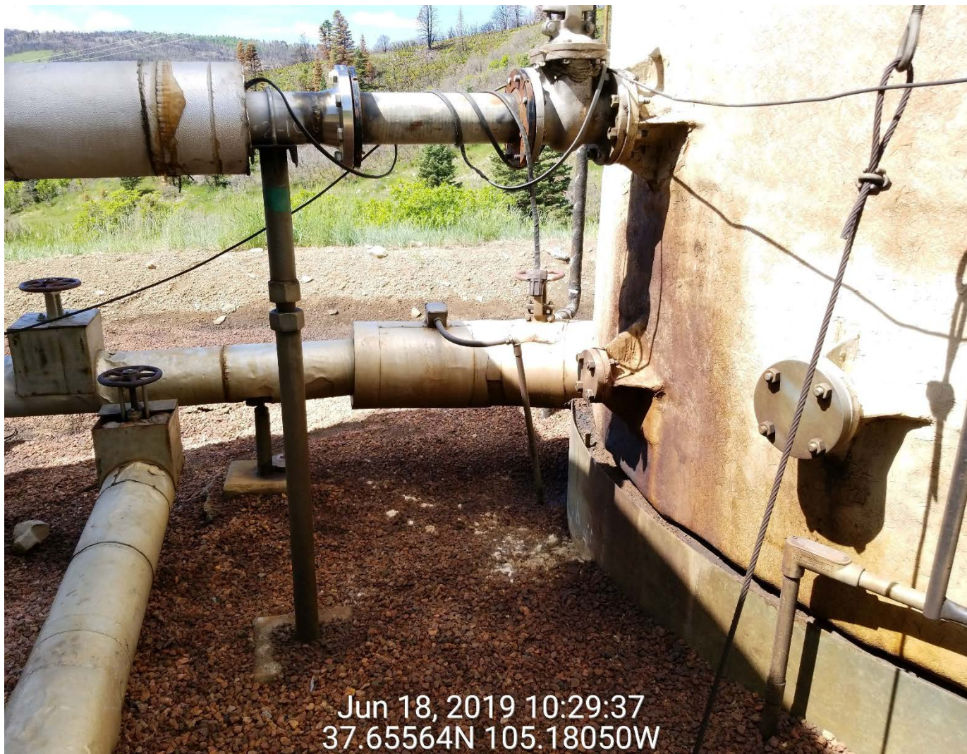
Source of leak and stained soil.
