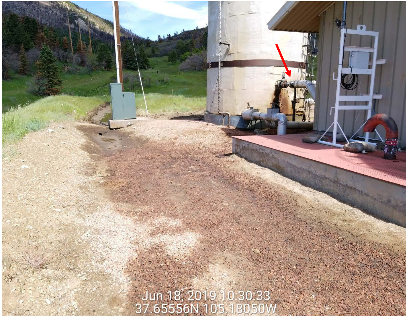
Source of leak and stained soil.
