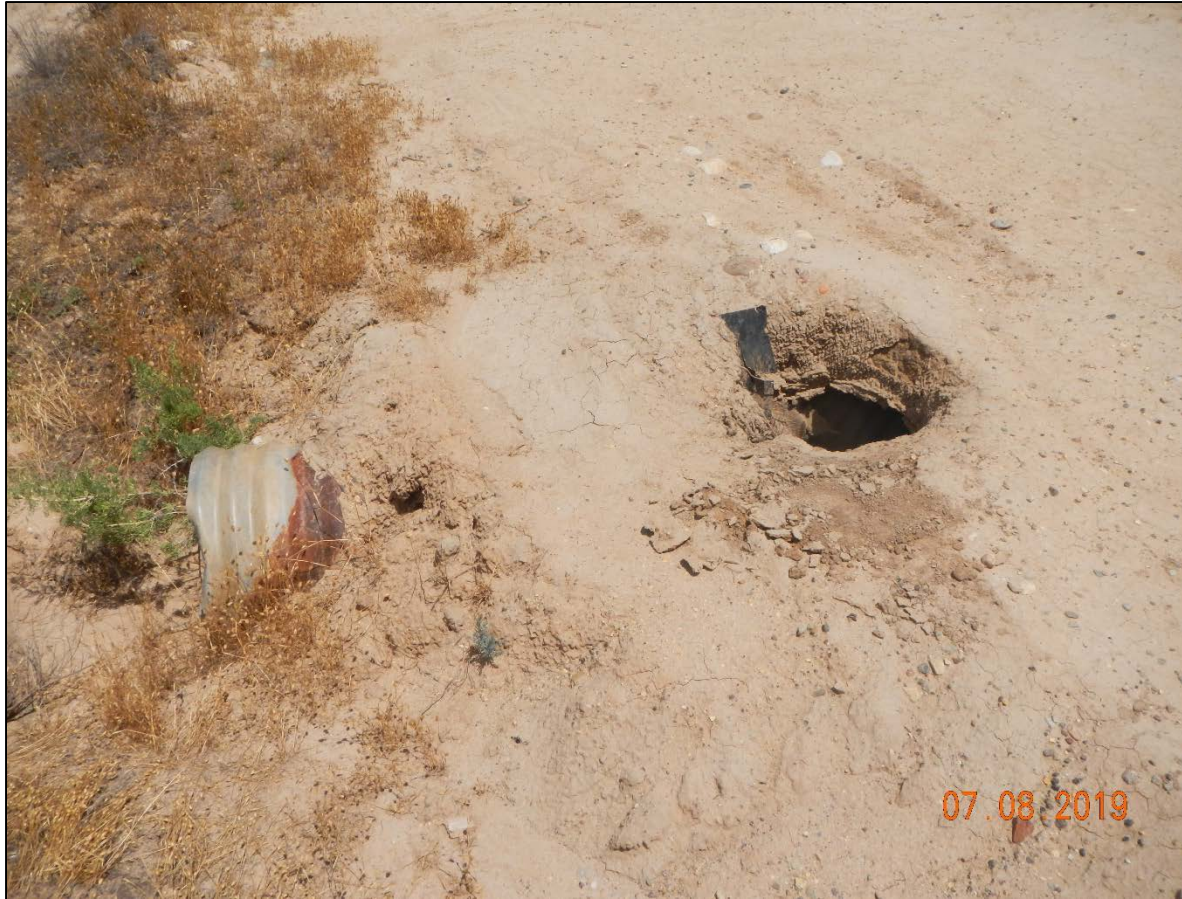
Hole in road over culvert.
