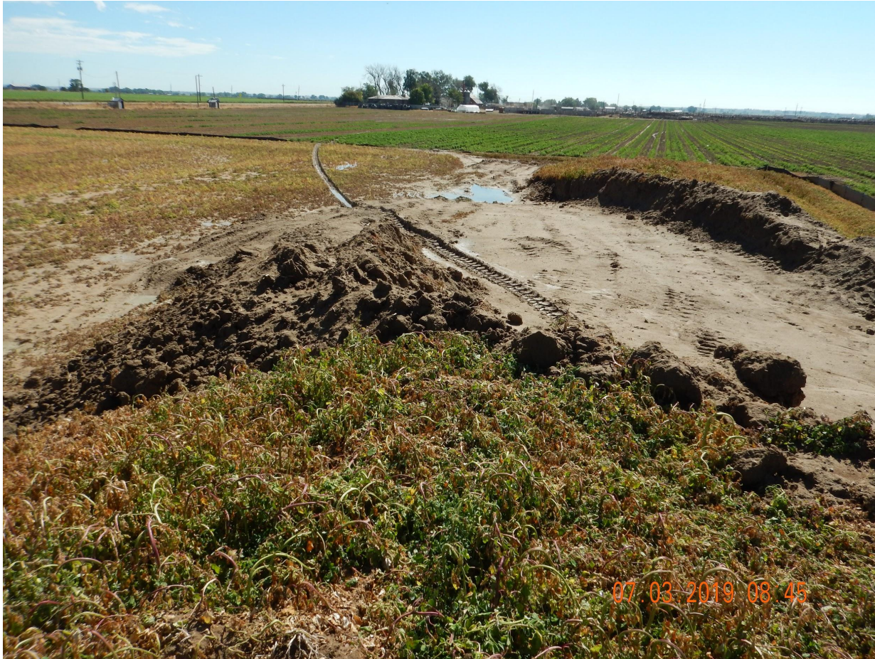
Photo 7. Photo taken from the eastern topsoil stockpile on July 3, 2019, facing East. Photo illustrates the Operator has failed to protect the topsoil per Rule 1002.c. Topsoil has been moved to allow the pivot irrigation system to travel through the well pad area.
