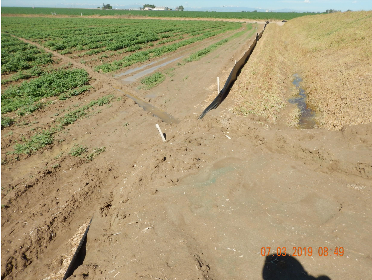
Photo 8. Photo taken from the eastern topsoil stockpile on July 3, 2019, facing West. Photo illustrates the Operator has failed to protect the topsoil per Rule 1002.c. and failed to maintain the perimeter stormwater BMPs.
