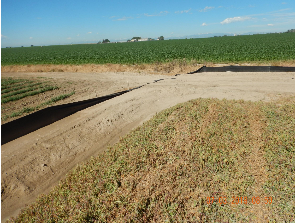
Photo 9. Photo taken from the western topsoil stockpile on July 3, 2019, facing West. Photo illustrates the Operator has failed to maintain the perimeter stormwater BMPs.
