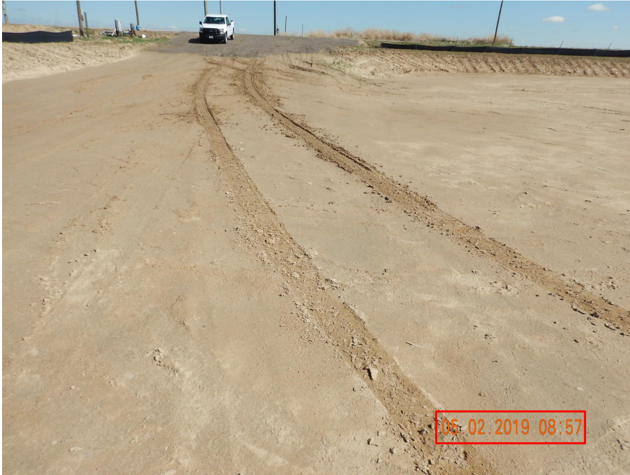
Photo 1. Photo taken from the northwestern well pad on May 2, 2019, facing North. Operator has not properly stabilized the well pad area to control for dust and erosion per Rule 1002.e.
