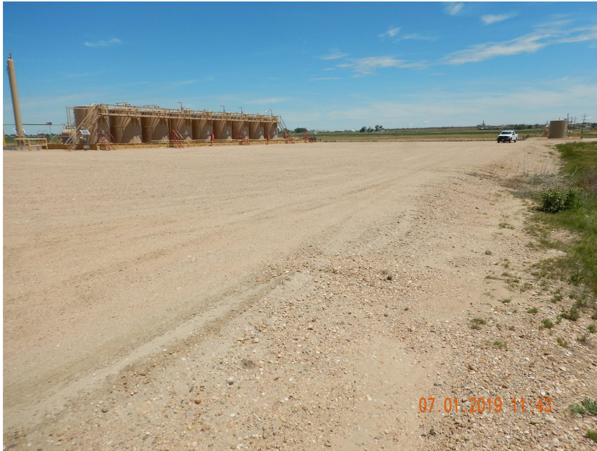
Photo 4. Photo taken along the southwestern location, facing East. Photo illustrates areas that do not appear to be needed for production operations; however, the Operator has not performed interim reclamation. Also, there was no apparent topsoil stockpile to facilitate future reclamation.
