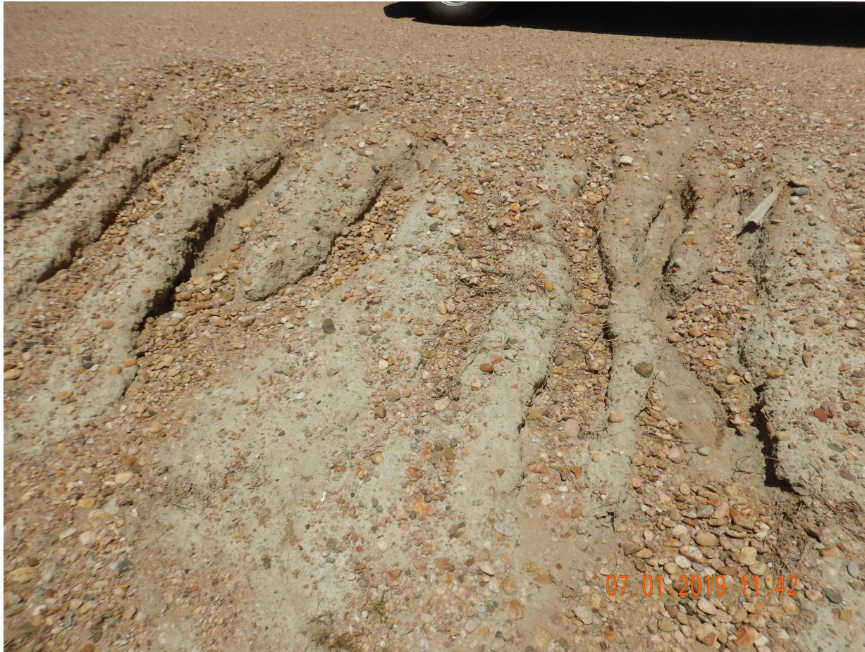
Photo 2. Photo taken from the southeastern location, facing North. Photo illustrates site degradation along the fill slope without stormwater erosion control BMPs.
