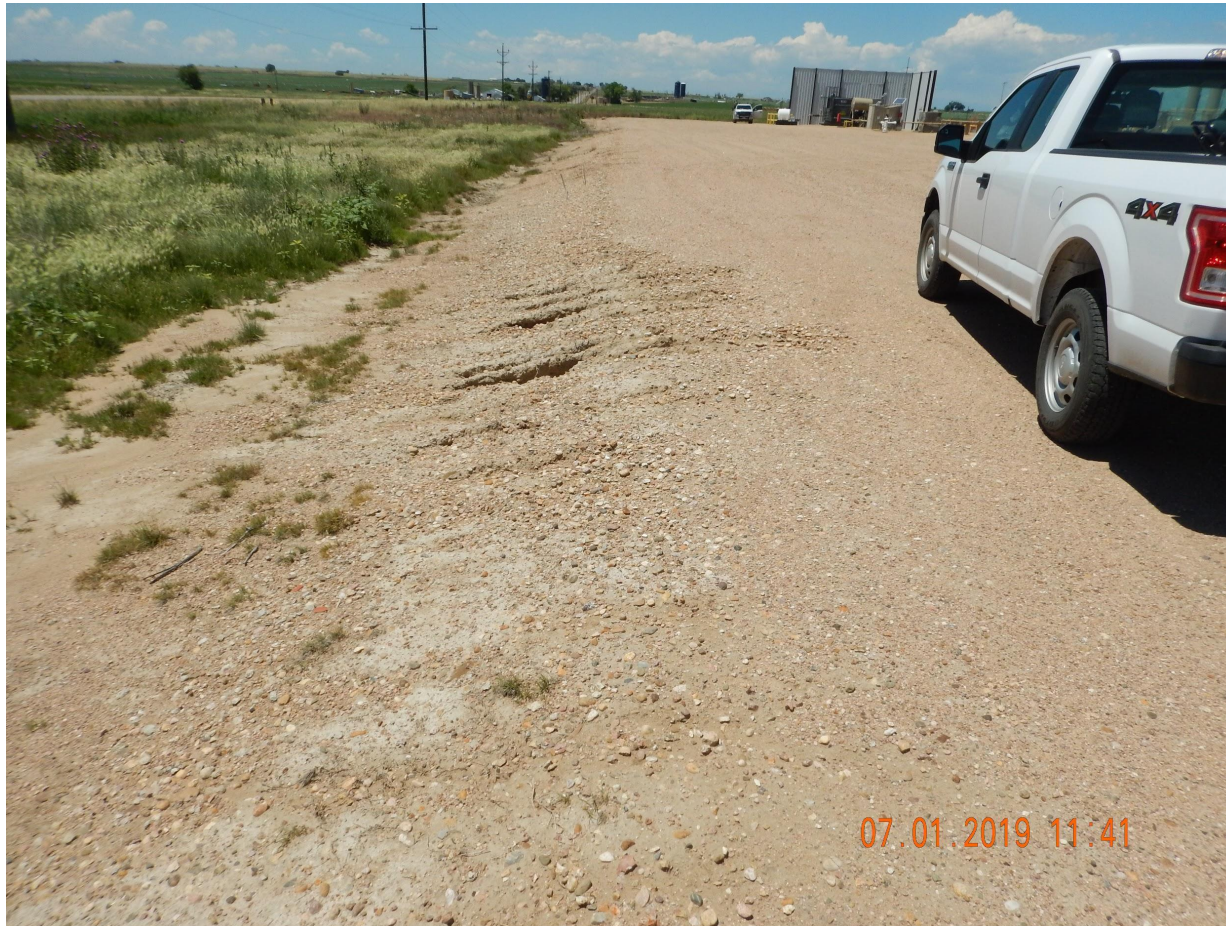
Photo 1. Photo taken from the southeastern location, facing West. Site degradation due to erosion was observed along portions of the perimeter of location without stormwater erosion control BMPs.
