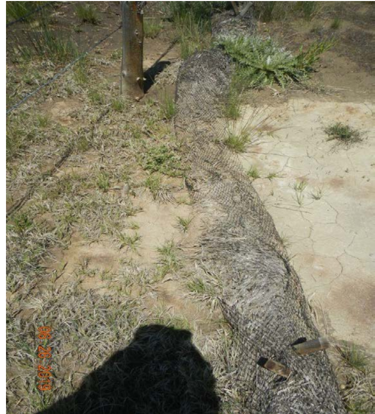
Photo#5: Compromised Wattle at site perimeter.
