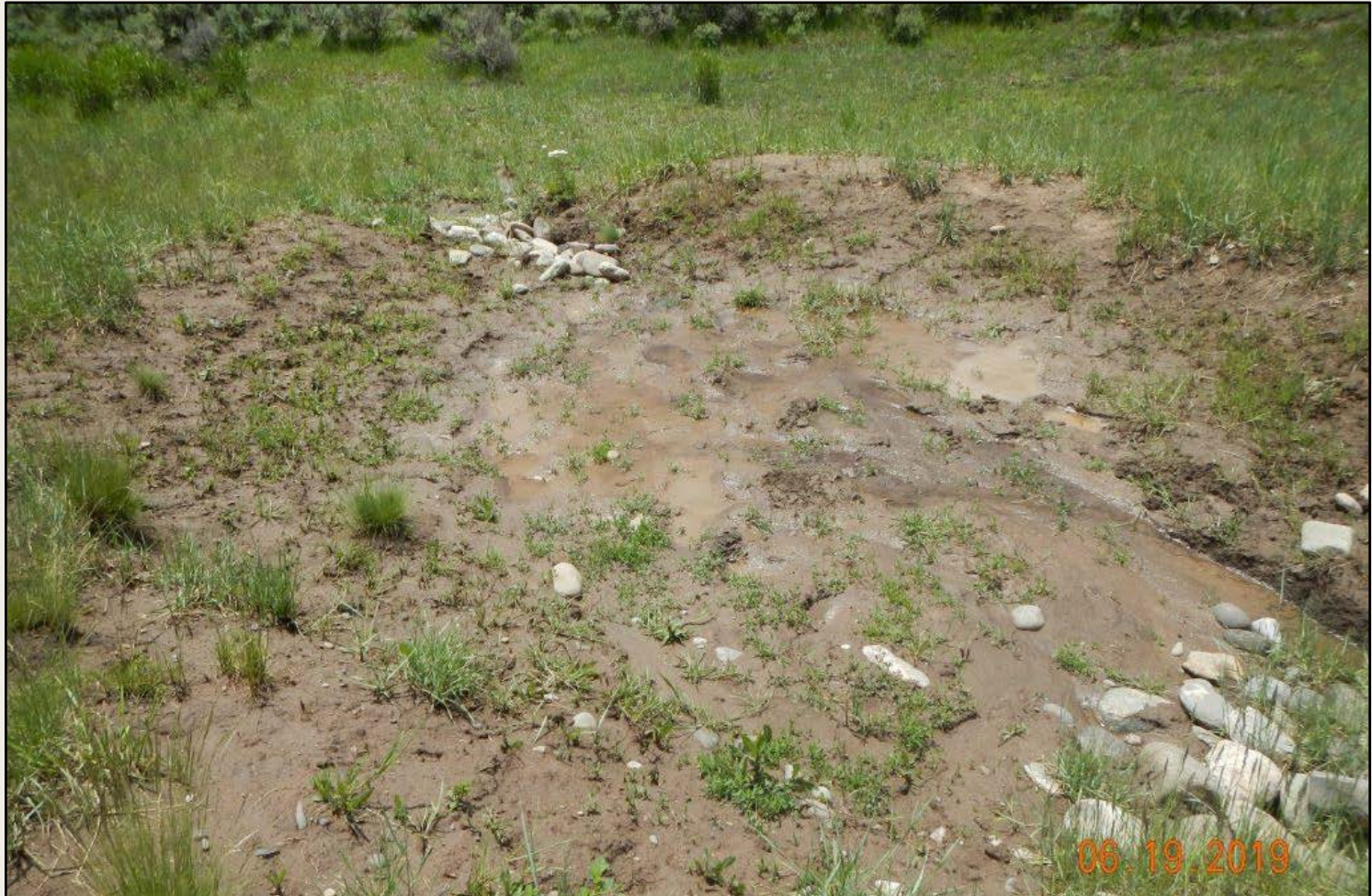
Photo 4. View of silt trap that is full of sediment.
