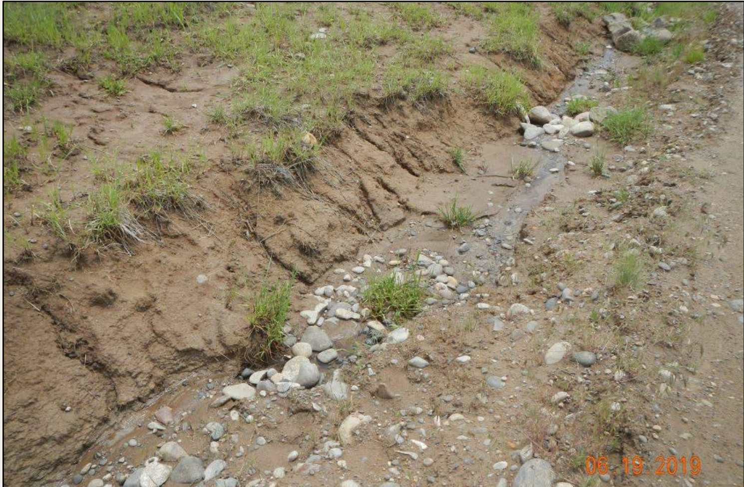
Photo 2. View of erosional channeling and unstabilized cut-banks along the access road.
