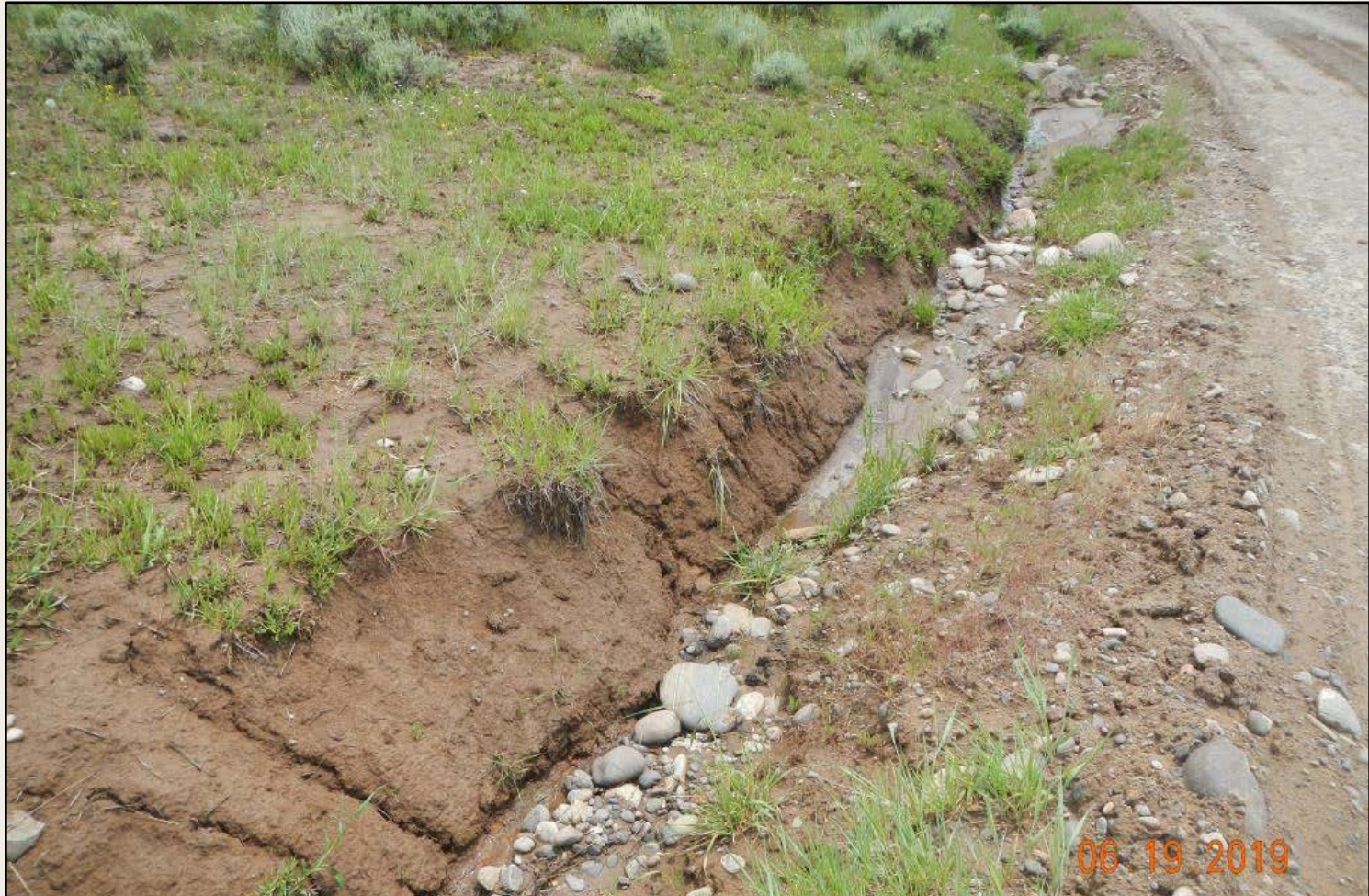
Photo 3. View of more erosional channeling and sediment deposition along the access road.
